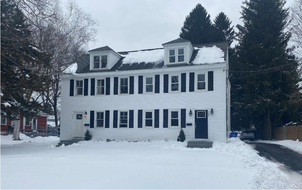
Photograph of the façade of 206-208 Concord Street
