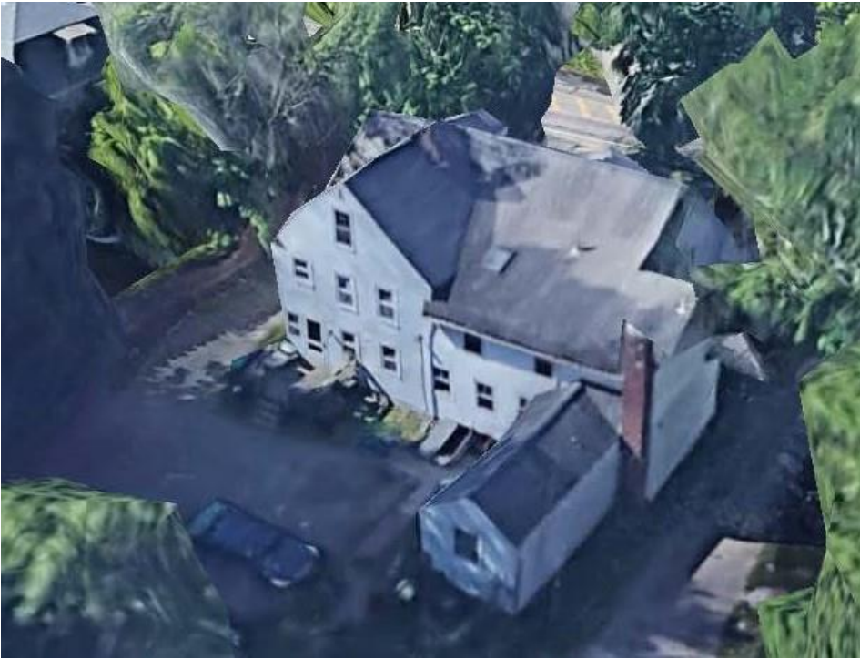
Google Earth image of the rear of 206-208 Concord Street
