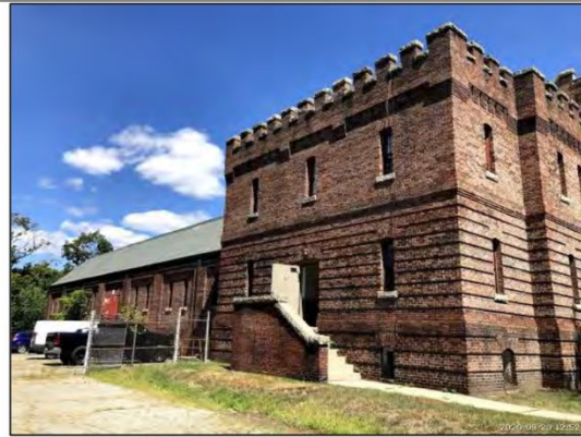
Photo 2: View of the western exterior of property building, facing east.
