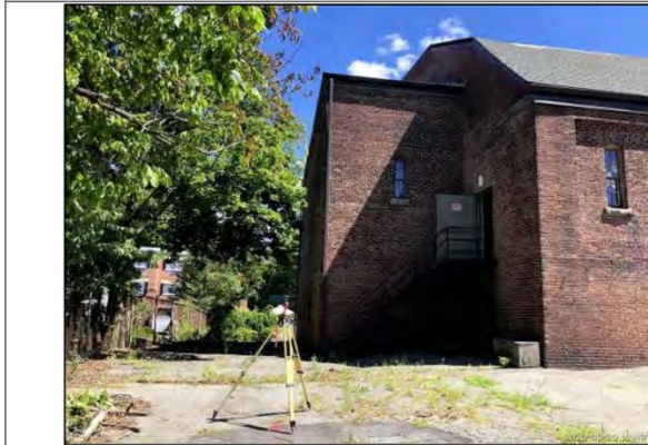
Photo 3: View of northern exterior of property building, facing east.
