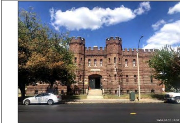
Photo 1: View of the southern exterior (front) of property building, facing south.
