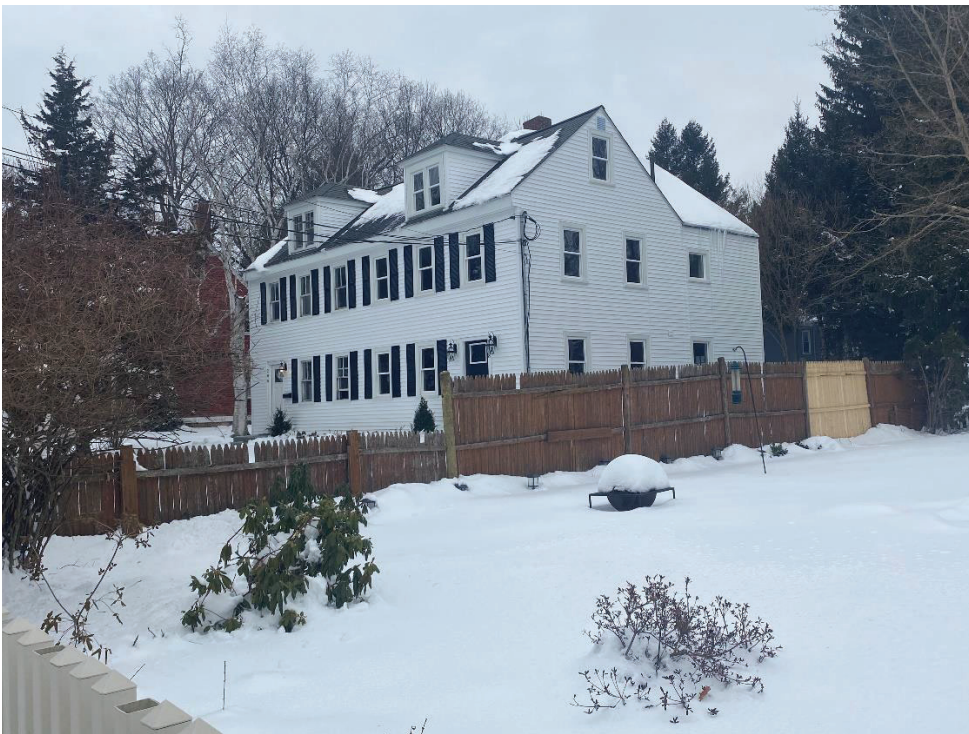
Photograph of the right side elevation and façade of 206-208 Concord Street
