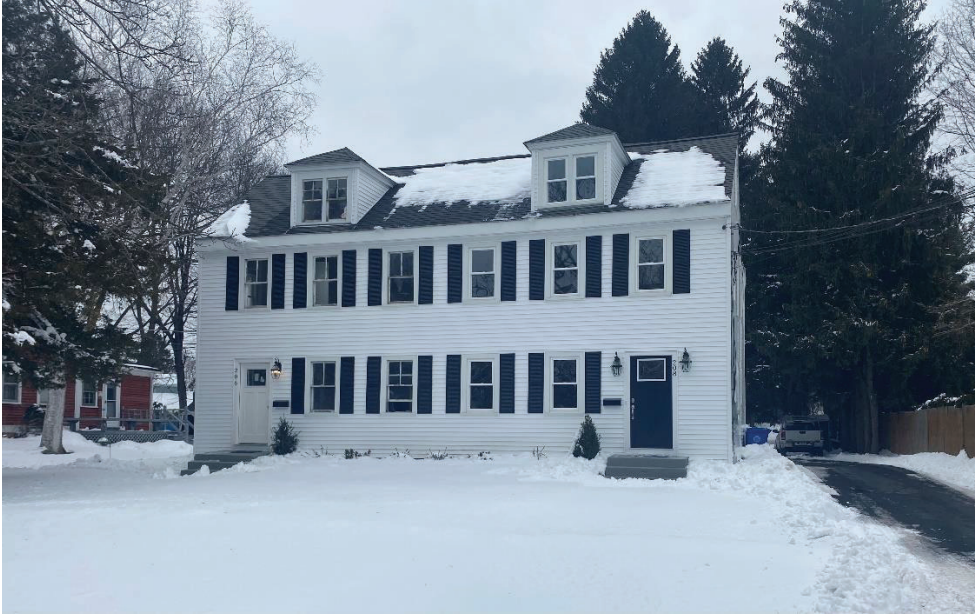
Photograph of the façade of 206-208 Concord Street
