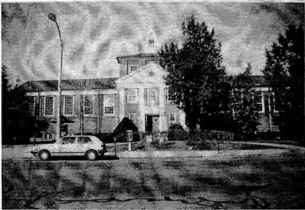
Figure 1: East elevation of Newtonville Branch Library, 1987. The landscaping of the site has changed considerably since then. The light fixtures on the limestone standards have also been changed. (Credit: Historic Newton)
