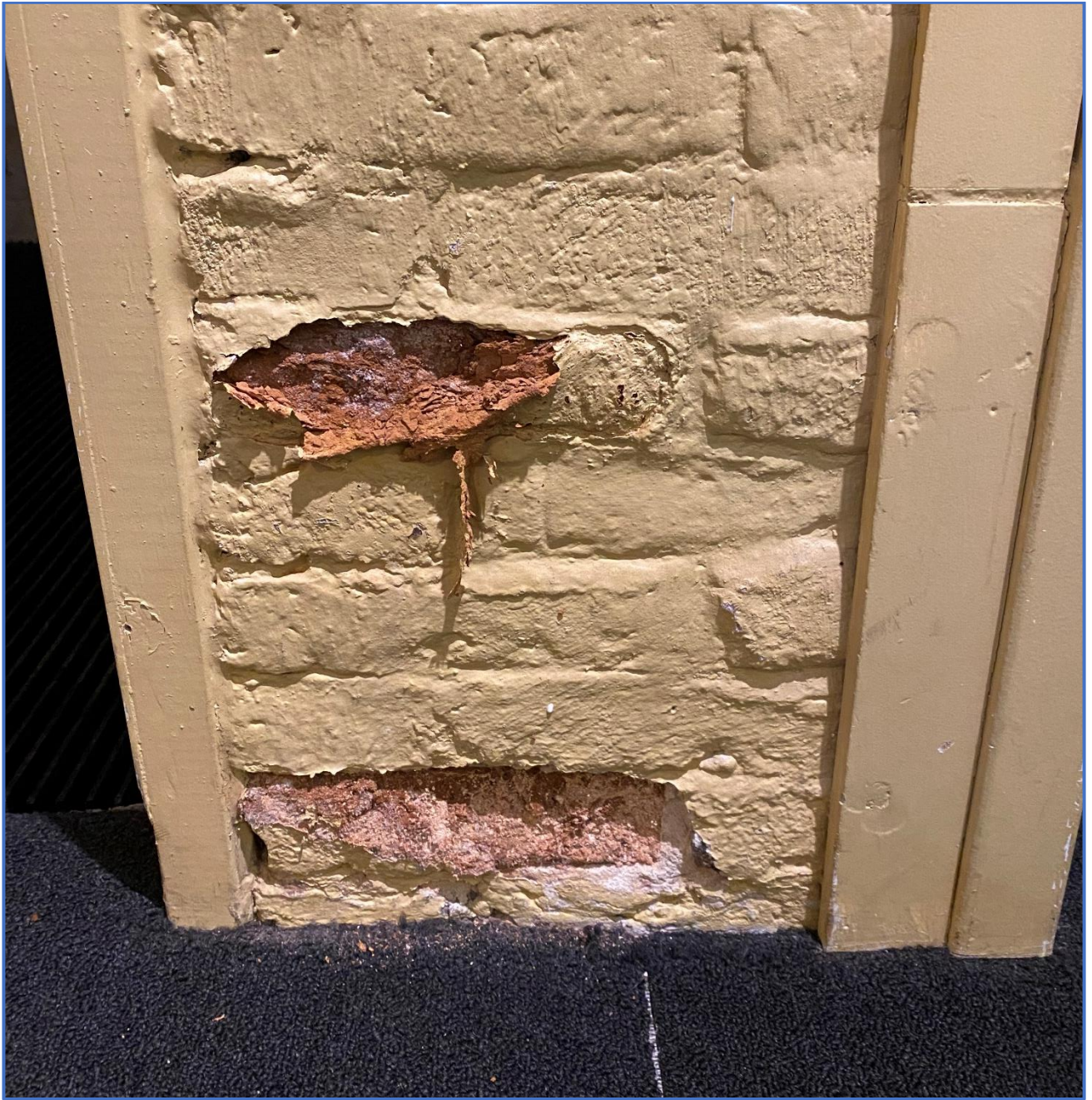
Foundation wall northwest
