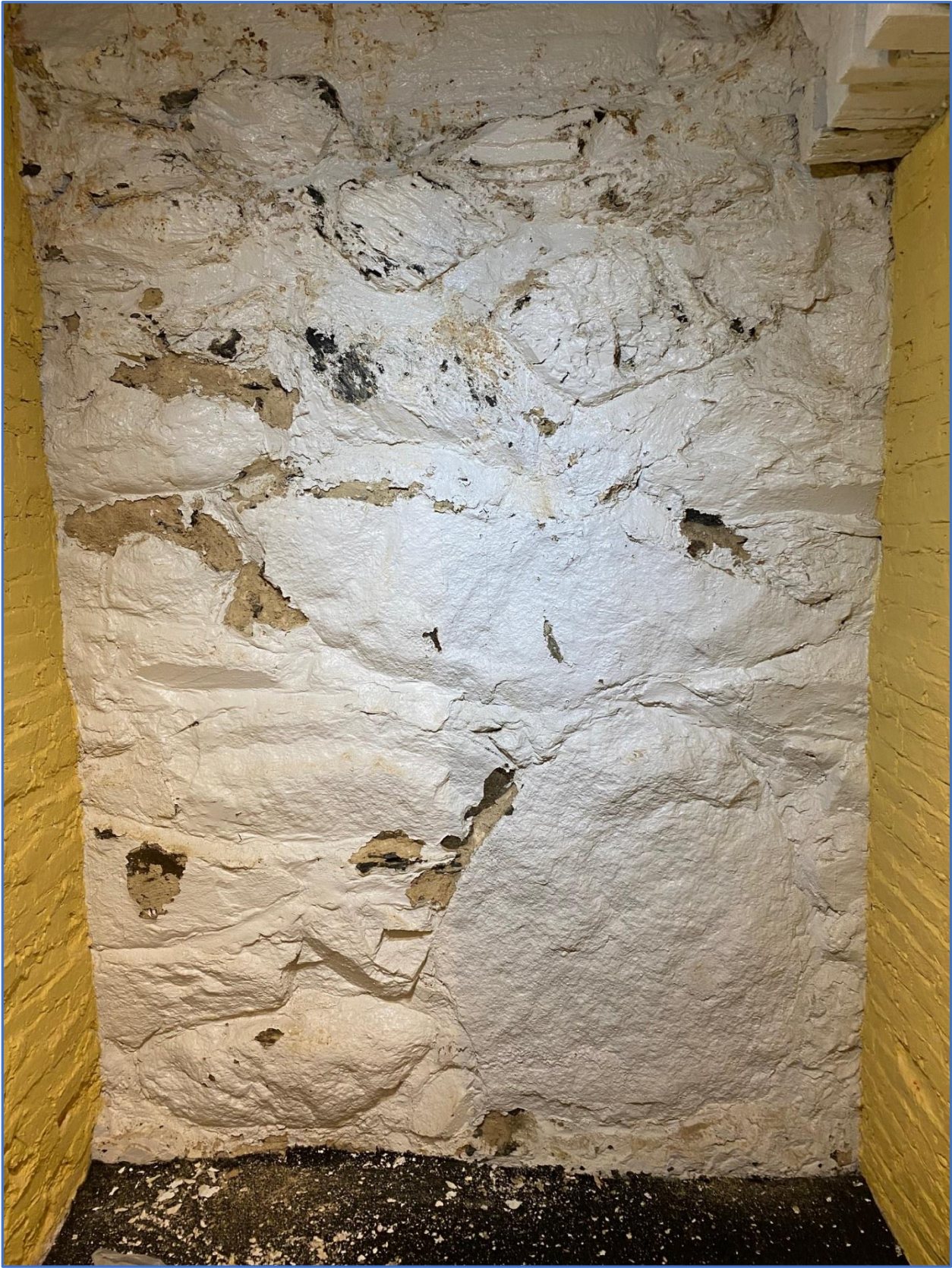
Fieldstone foundation wall, west.
