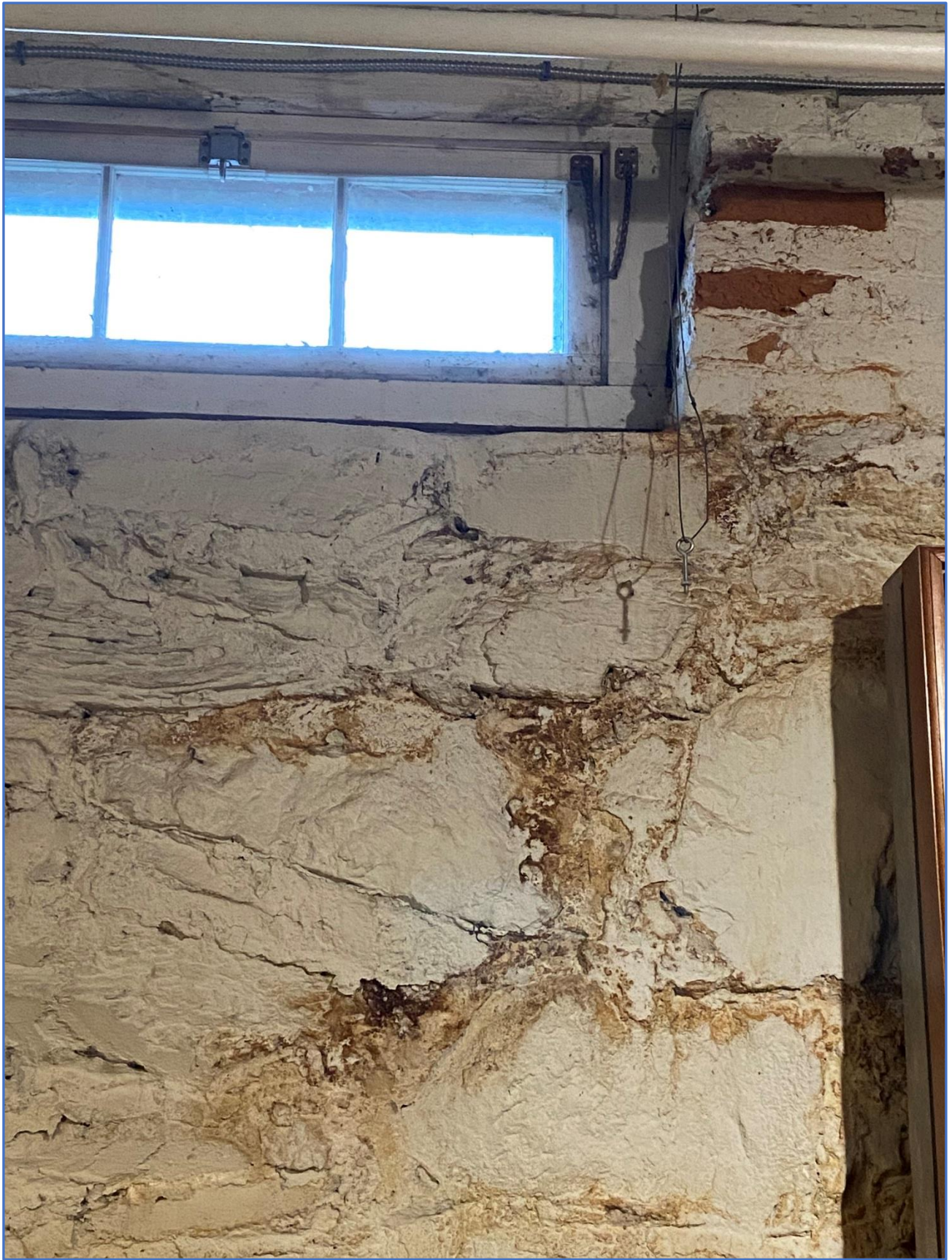
Foundation wall south
