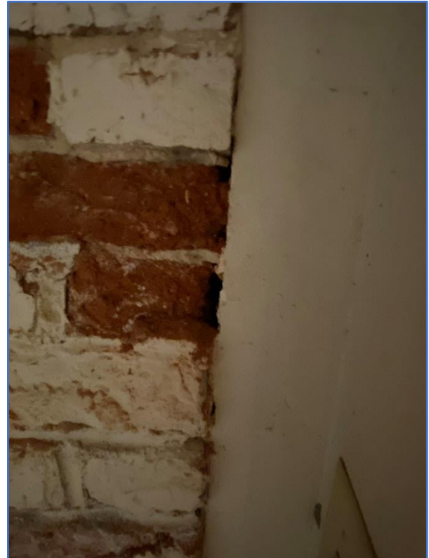
Foundation wall NE closet
