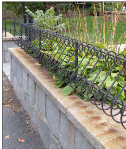
This stone wall is topped by a decorative iron fence with an S-shaped profile.
