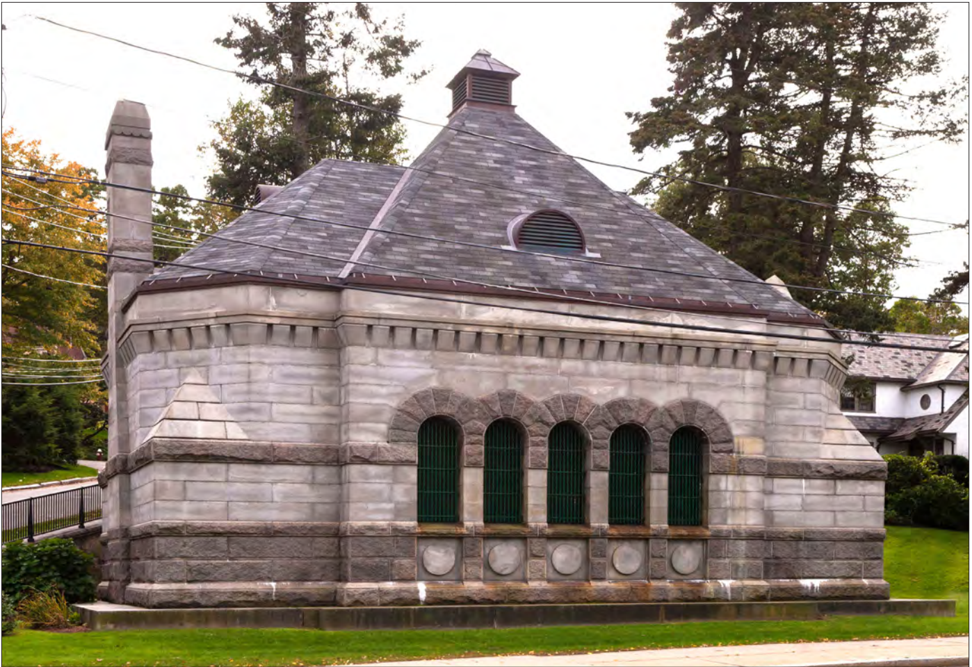
The Sudbury River Conduit Gatehouse is a key feature in the Chestnut Hill Historic District.
