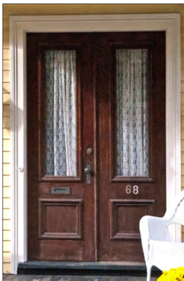
Paired wood doors, which often include glass lights, are typical of Victorian period buildings.
