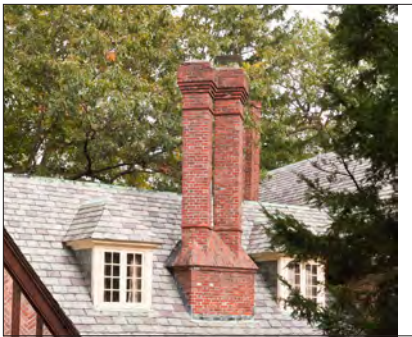
Chimneys can range from simple forms to the complex as seen in this paired-shaft, corbelled brick chimney.
