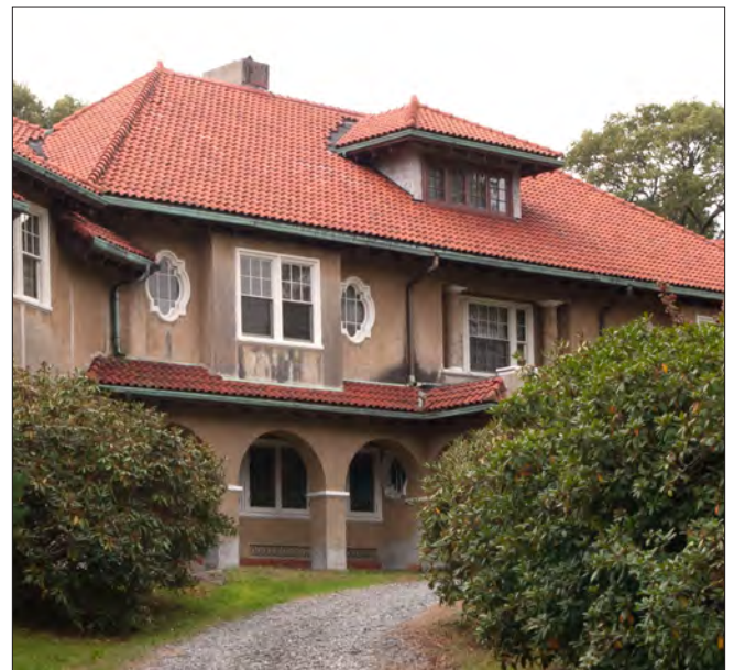
Tile roofs can often last as long as slate roofs, and contribute greatly to the character of buildings such as this historic home.
