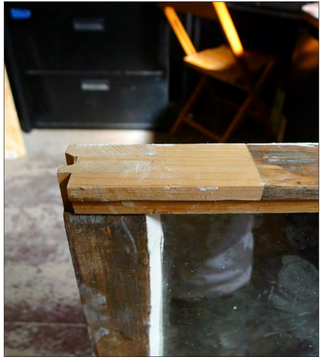
One of the advantages of historic wood windows over modern prefabricated units is repairability. This photo demonstrates a dutchman repair at the corner of a historic wood window. Also note the new glazing putty.
