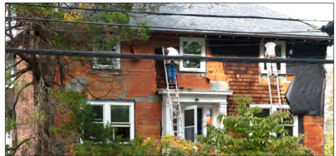
When repair is not possible, the NHC/HDC encourages in-kind replacement.
