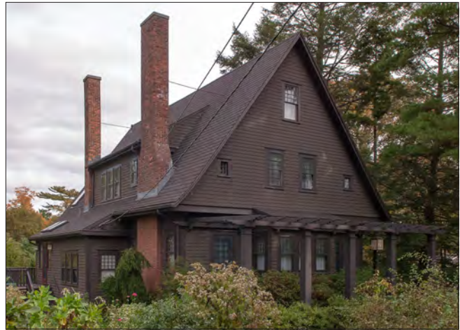
Overall roof form, detailing and historic roof features are an important element of many of Newton's historic homes, such as this example in Auburndale.
