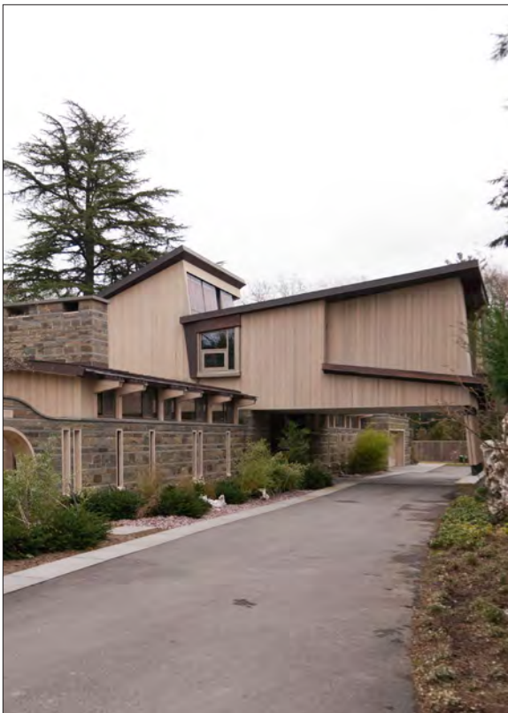
This Contemporary home in Chestnut Hill features irregular geometric shapes, varied window openings and a combination of exterior cladding materials.
