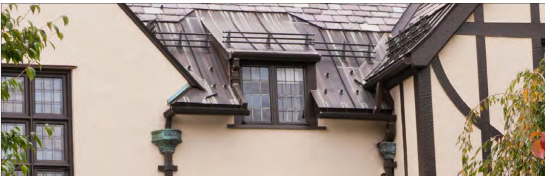
Snow guards come in a variety of types and styles, as seen on this roof. Also note the standing-seam metal roof with copper gutters, downspouts and decorative copper scuppers.
