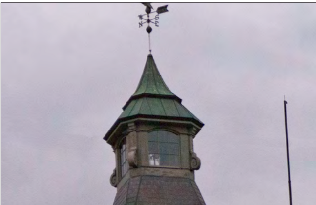
Metal standing-seam roofs were popularized in the mid-19th century. Decorative or unusually shaped roof elements, such as this cupola, were often covered with metal roofing.
