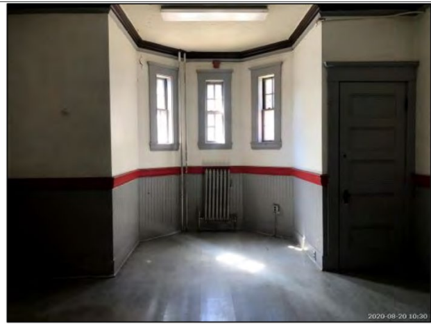
Photo 11: Ground level room, typical.
