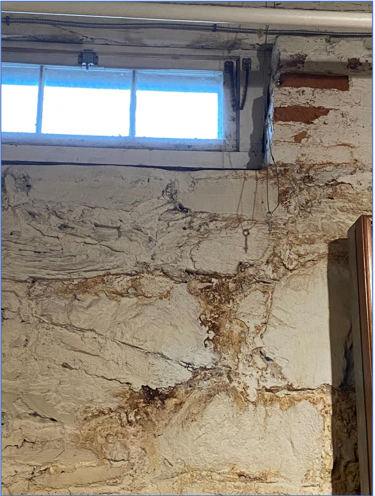
Foundation wall south
