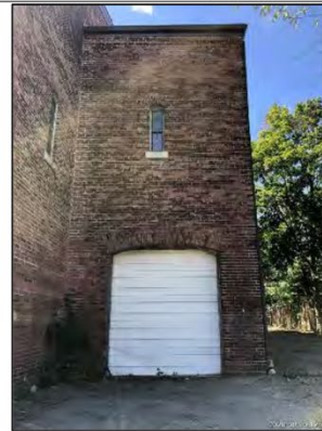
Photo 4: View of entrance to garage, along north of building.
