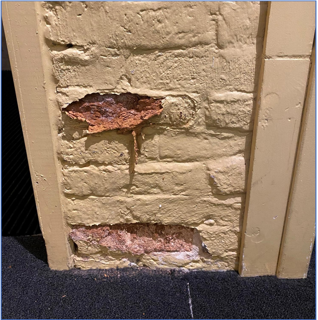
Foundation wall northwest
