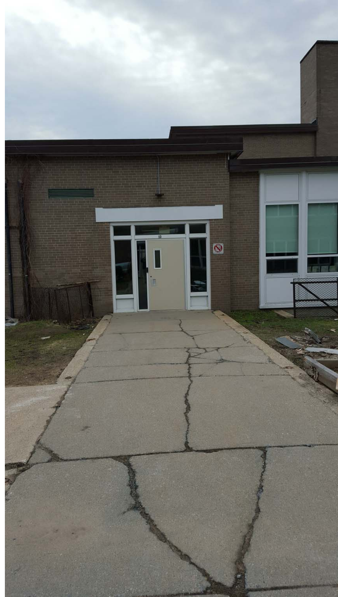
② EXISTING WALKWAY & EAST FACADE
