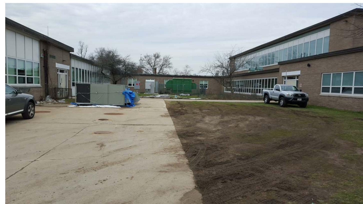
⑥ EXISTING COURTYARD LOOKING SOUTH (MODULAR SITE ON LAWN TO RIGHT)
