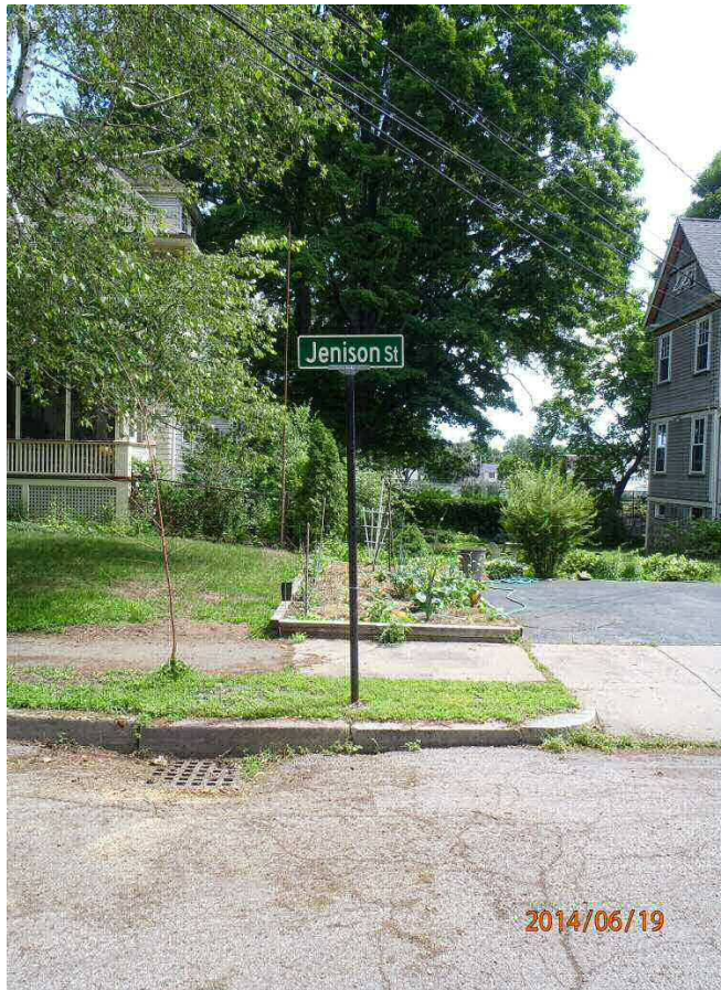
Catch basin located at the intersection of Judkins Street and Jenison Street
