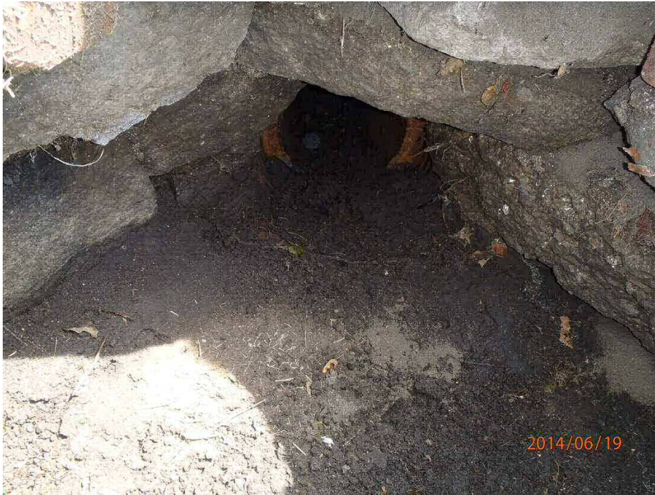
6-inch Drain Pipe Connection at Manhole at Pellegrini Park
