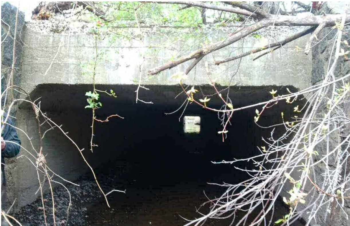
Upstream Side of Upland Ave. Culvert
