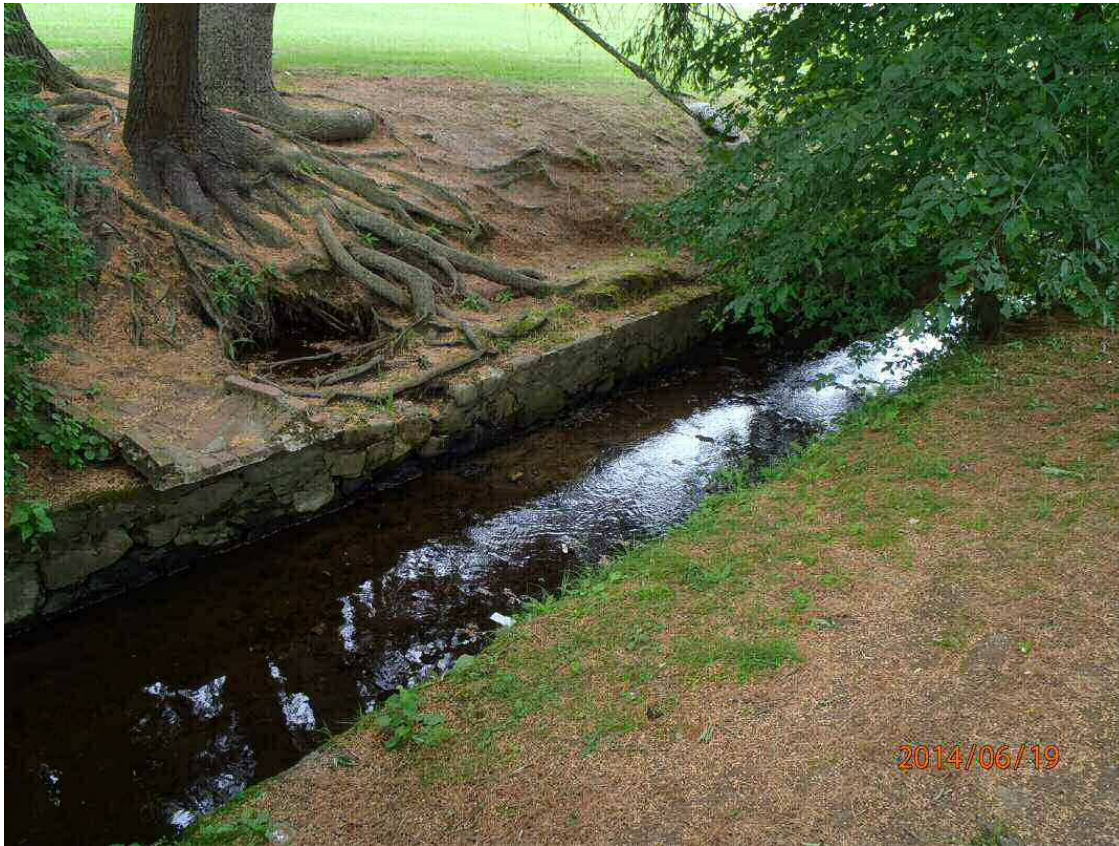
Sinkhole Near Hammond Brook from Underdrain Flow
