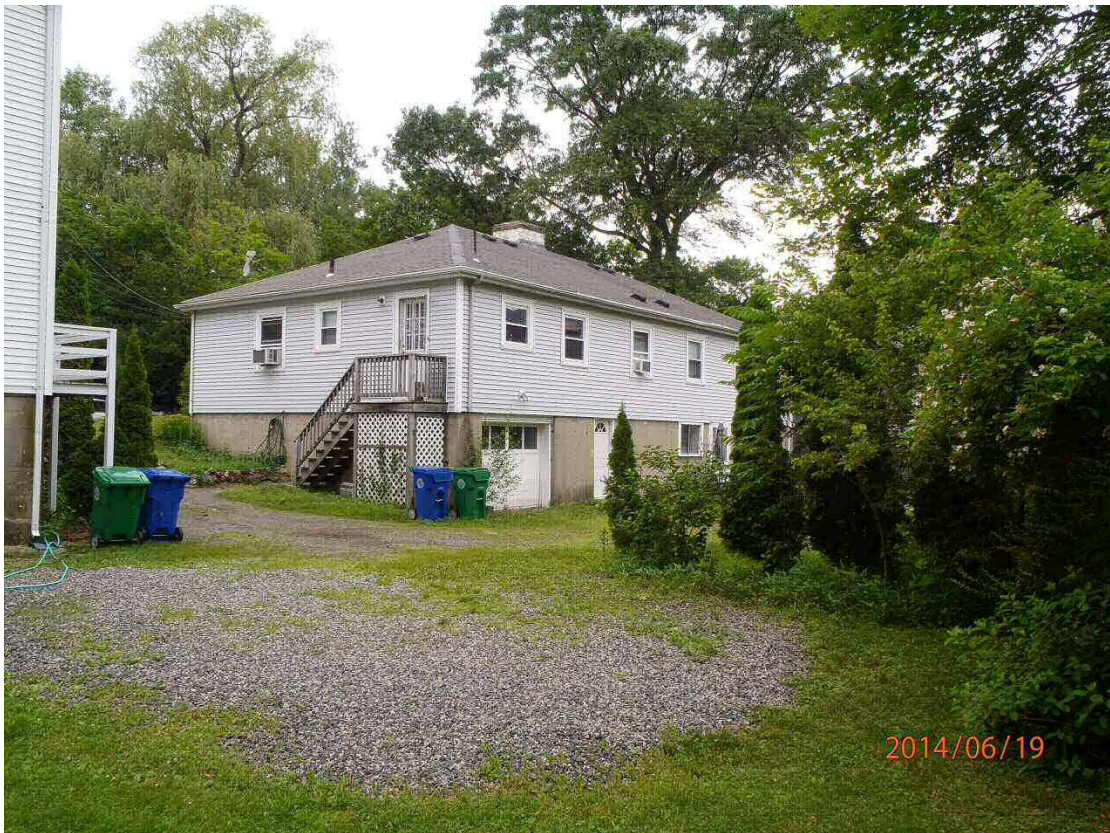
Rear Yard of #62 Beaconwood Road Looking Towards the Road
