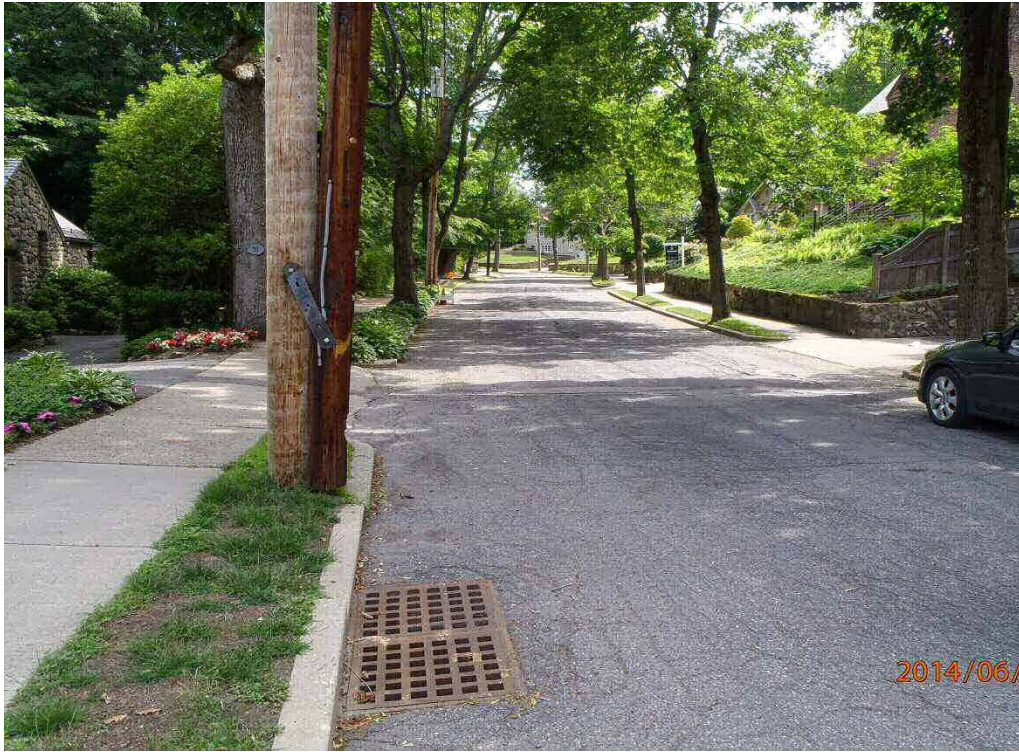
At Double Catch Basins Looking North on Oldham Road
