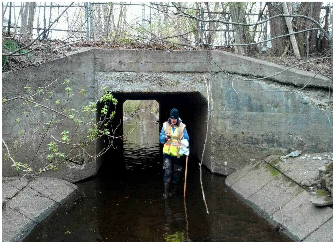
Downstream Side of Dedham Street Culvert
