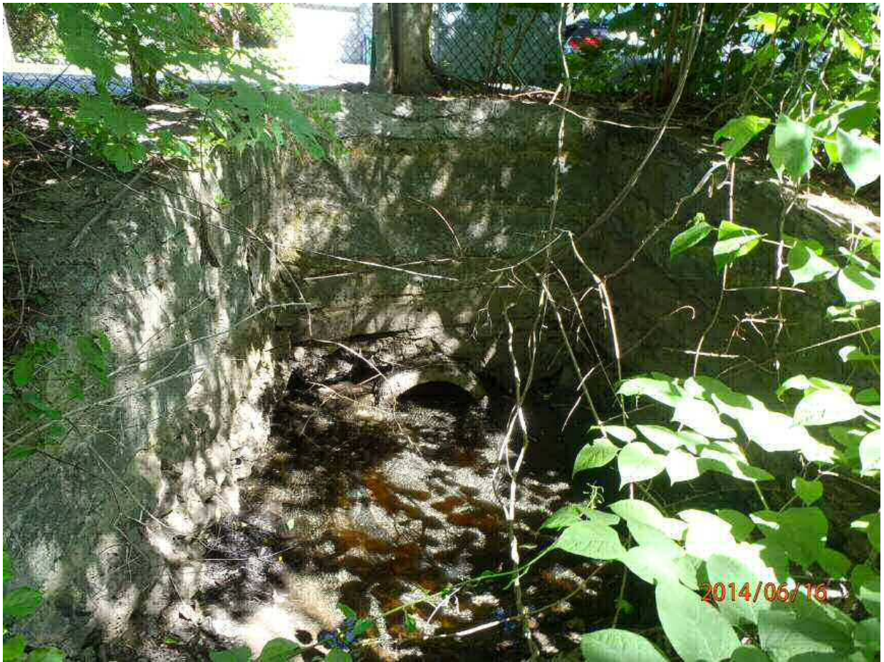
Wayne Road Outfall
