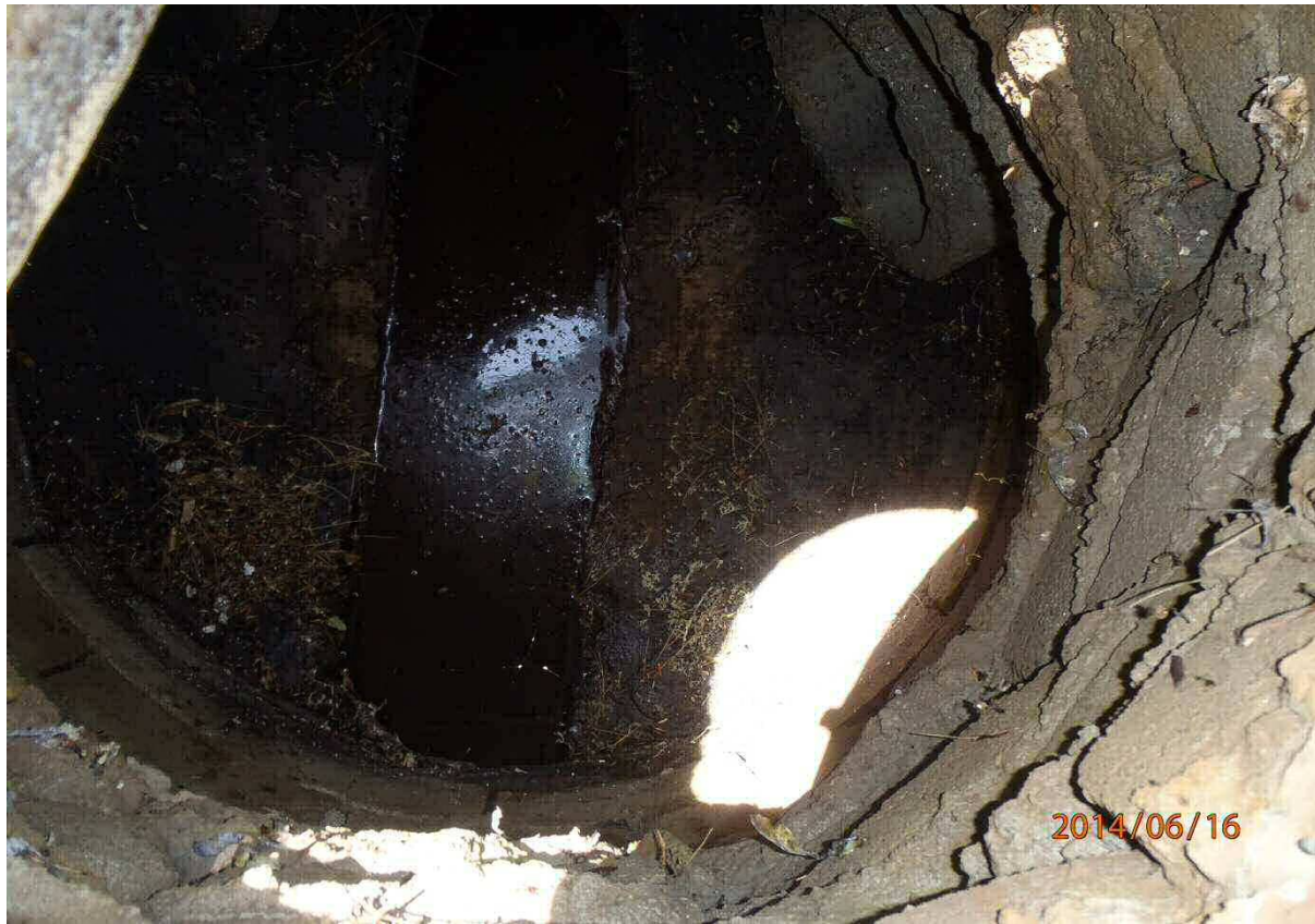
Drain Manhole on Dedham Street Upstream of Dedham Street Culvert
