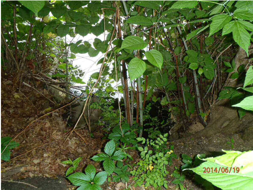
Culvert Under Footpath Near Beaconwood Road
