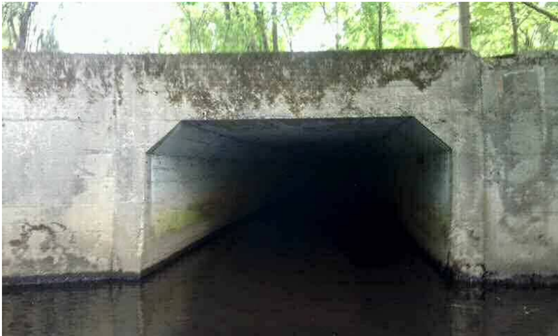
Upstream Side of Culvert for Saw Mill Brook Under Hollywood Drive
