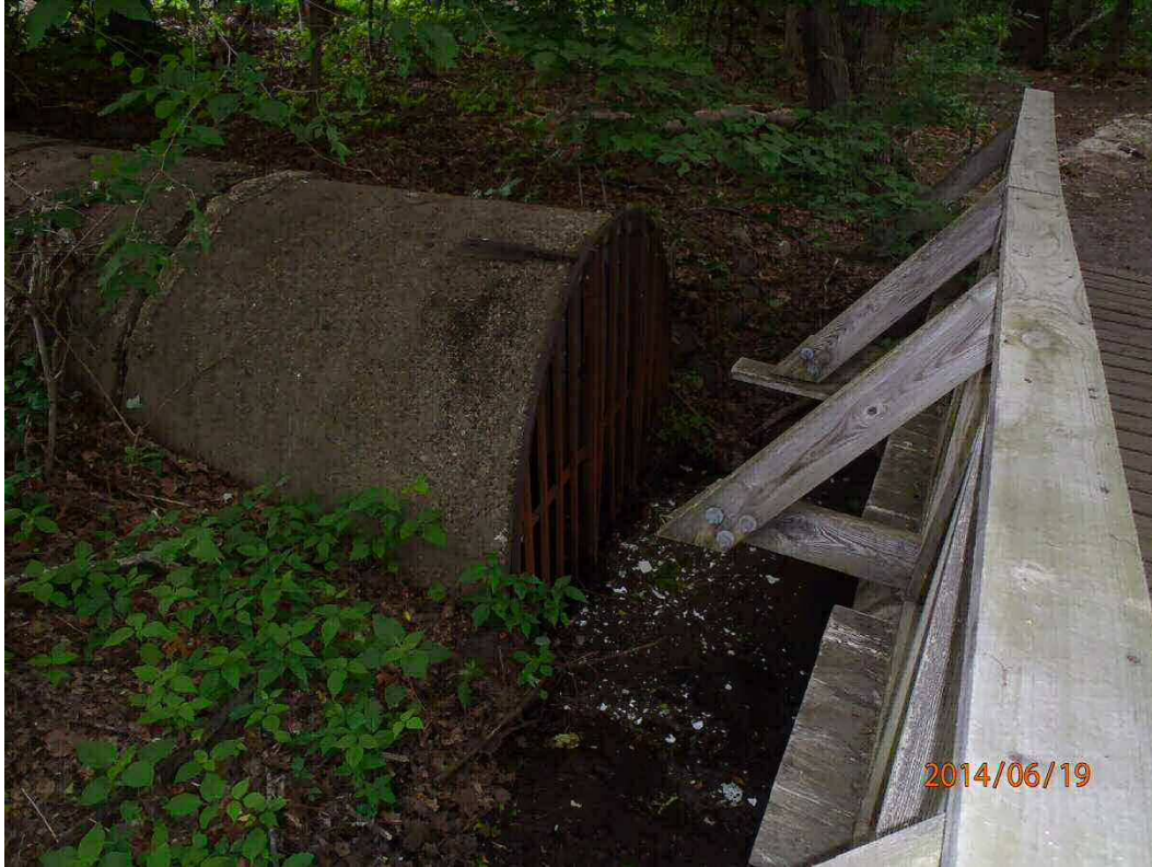
Inlet to 66-inch Culvert Underneath the Zervas School
