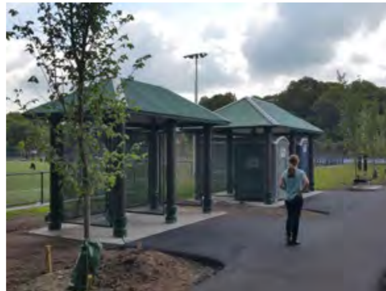
Bathroom Enclosure Structure
