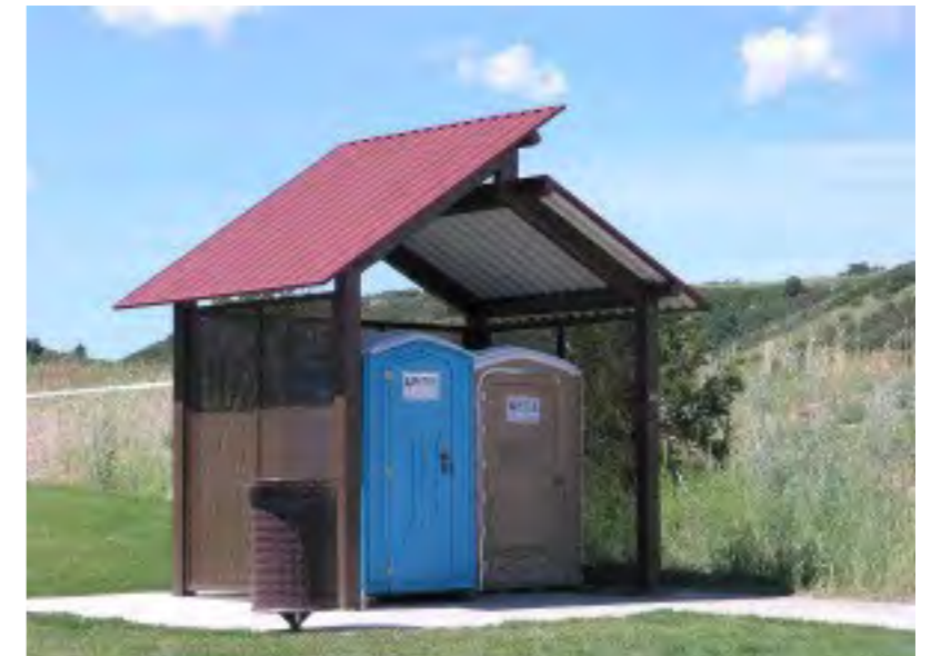
Bathroom Enclosure Structure
