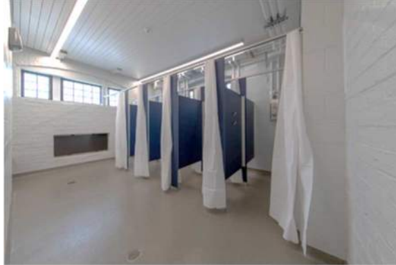
Shower Stalls Dry and Wet Sections
