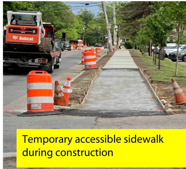
Temp. Asphalt ramp & temp cross walk painted
