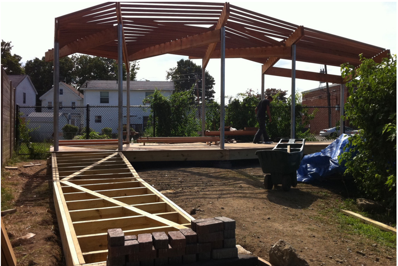
Construction in process
