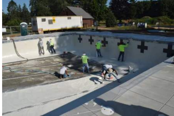
White Plaster with Tile Wall Targets and Racing Lines
