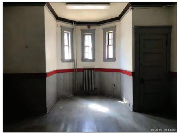
Photo 11: Ground level room, typical.
