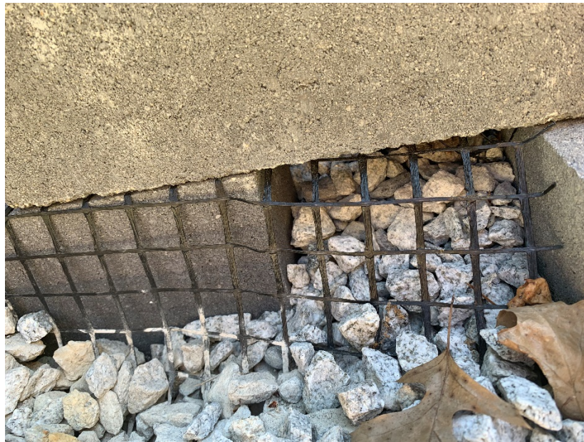
The fiberglass geogrid seen between the 3 rd & 4 th course of blocks
