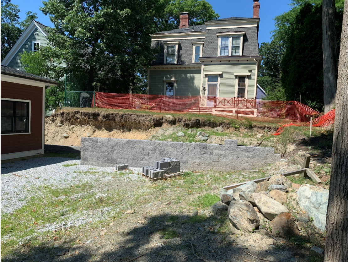
View of wall constructed to date looking west.
