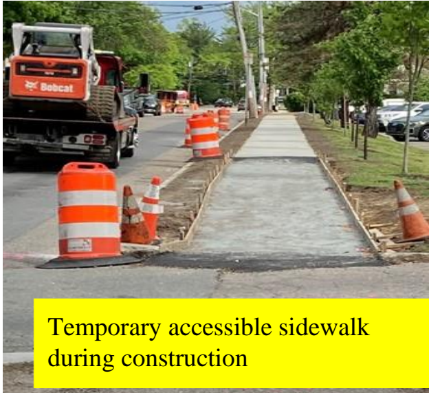
Temp. Asphalt ramp & temp cross walk painted
