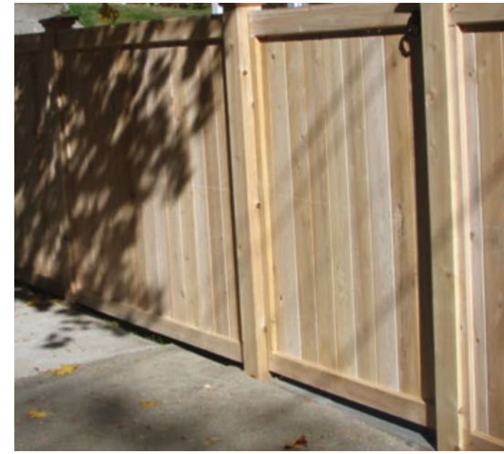
GATE AROUND TRASH Universal Style White Cedar Fencing 4' High on Three Sides 3 Gates on Front Per Layout Plan
