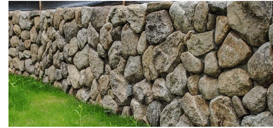
NEW ENGLAND FIELDSTONE RETAINING WALLS All Proposed Retaining Walls Made of New England Fieldstone Walls 16". Height varies. See Elevations. Raked Mortarless Joints. No Cap.
