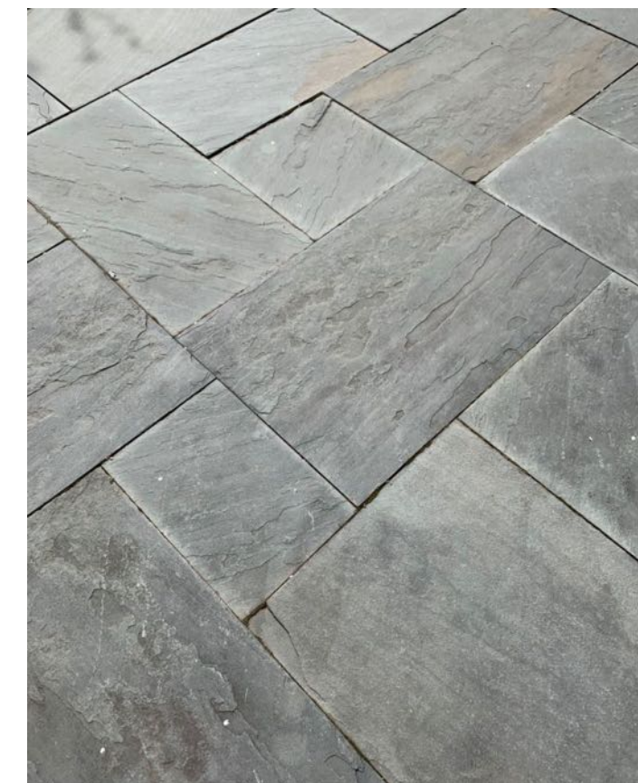
BLUESTONE LANDINGS and STEPS All Landings All Blue Natural Cleft Bluestone in Random Rectilinear pattern Thermal Bluestone Treads for Borders and Treads of Stairs All Steps 7.5" with 1% Pitch, except for step down to first landing from front door. Meet existing elevation of landing.
