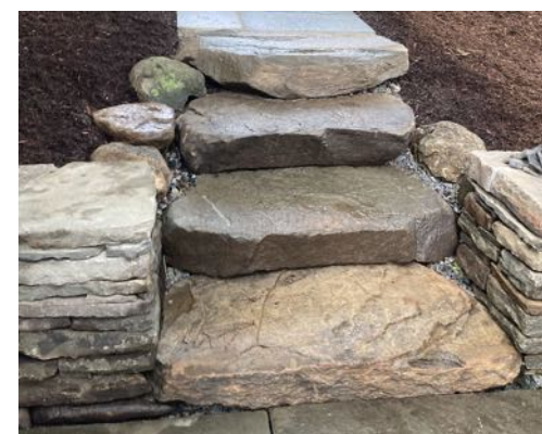
FIELDSTONE STEPS 3 x Fieldstone Steps 5-6" Risers, +/- 36" Wide TYP
