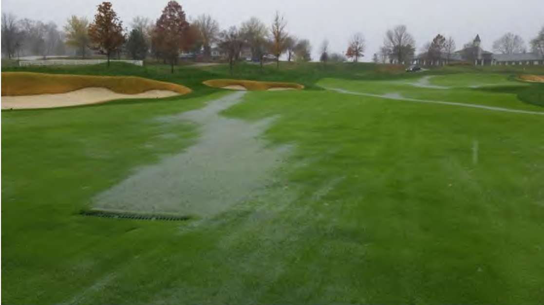
Figure 4- Channel Drain at Valhalla Golf Club
