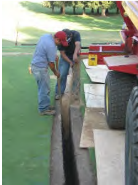
Backfilling trenching with sand
