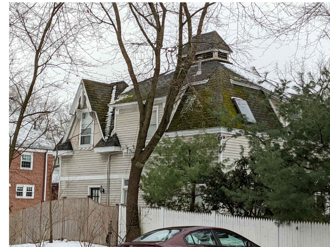
EXISTING SIDE FROM NEIGHBOR
