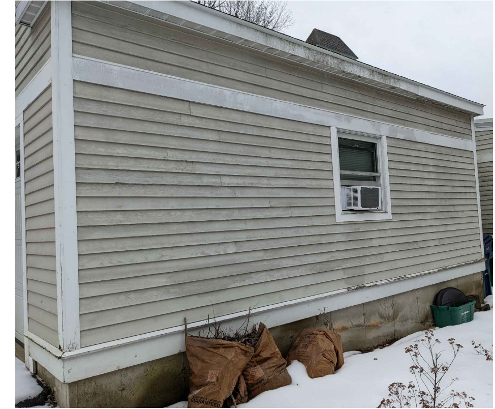
EXISTING SIDE OF GARAGE
