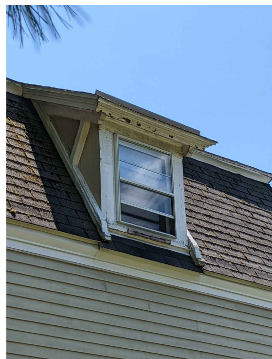
EXISTING FRONT DORMER WINDOW
