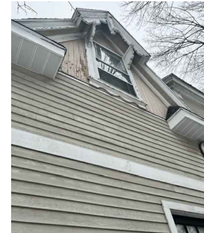
EXISTING SIDE WINDOW
