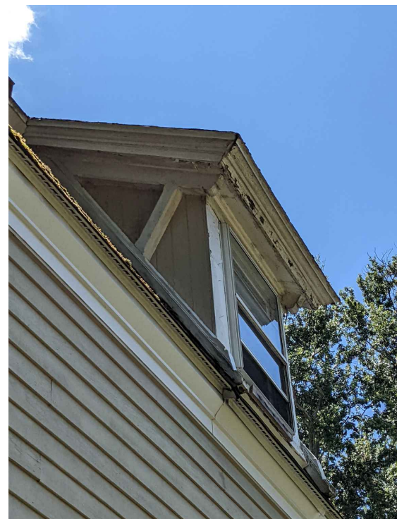
EXISTING FRONT DORMER WINDOW
