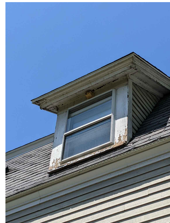
EXISTING FRONT DORMER WINDOW
