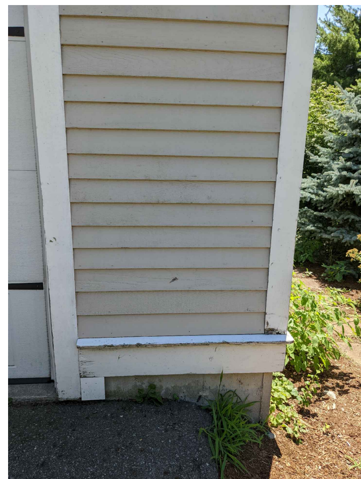
CONDITION AT SIDE OF GARAGE
