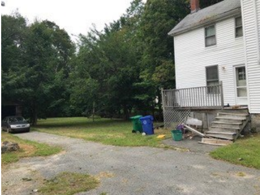
Photograph 1: Existing residential structure, driveway, and shed/garage on the site.
