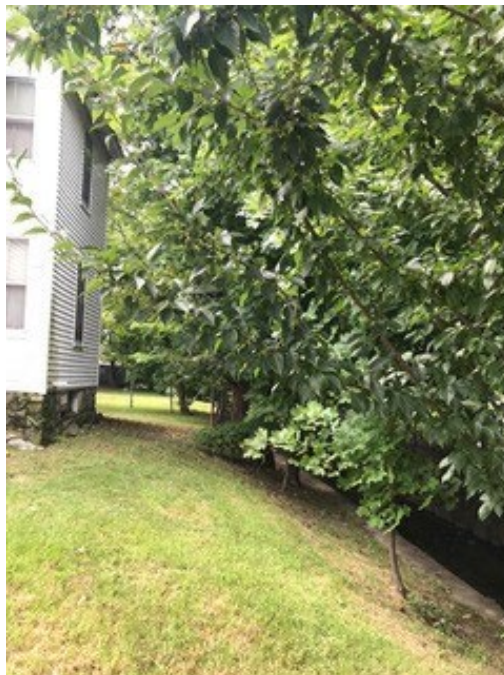
Photograph 2: Existing structure and proximity to Cheese Cake Brook.
