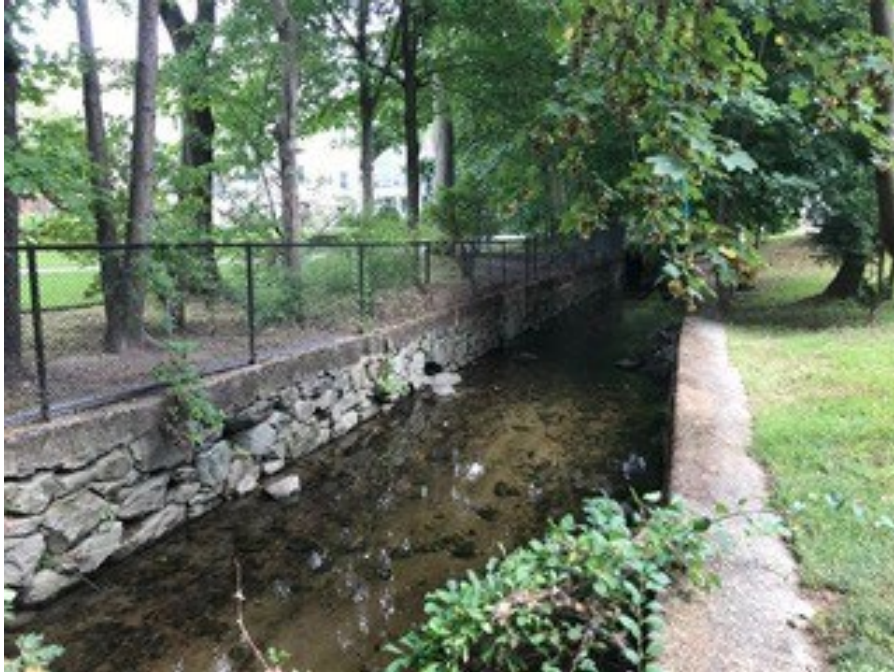
Photograph 3: Cheese Cake Brook within the constructed stone/concrete Banks.
