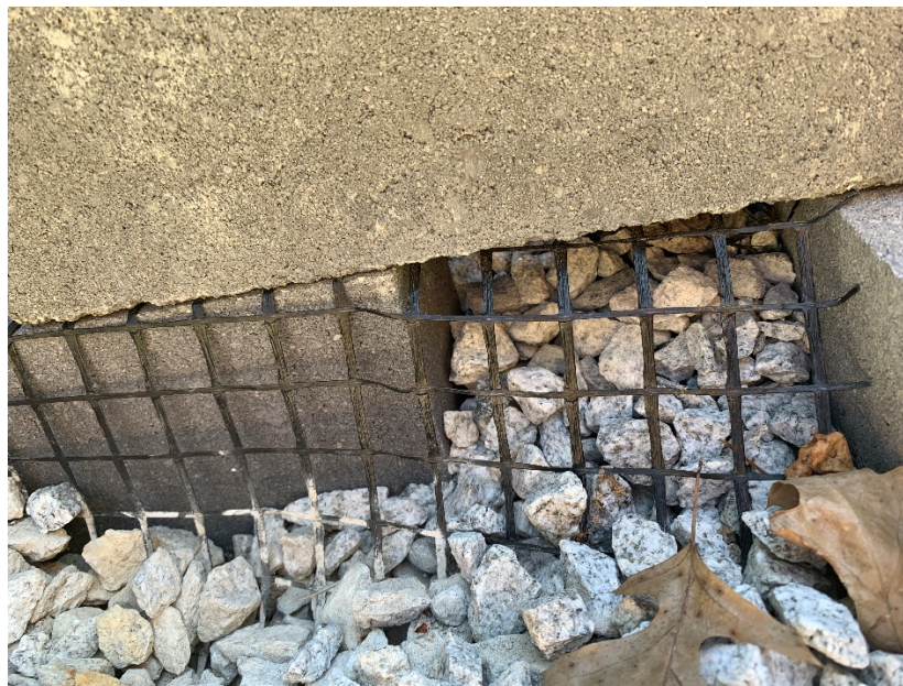
The fiberglass geogrid seen between the 3 rd & 4 th course of blocks
