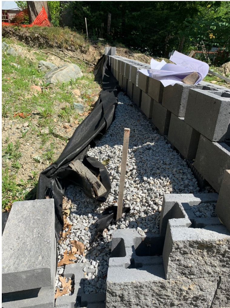
The black filter fabric & crushed stone for proper drainage
