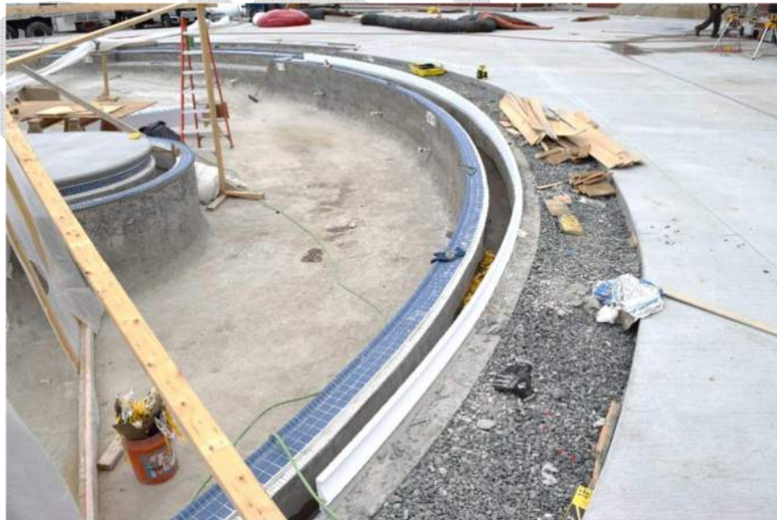
Formed Pool Gutter at the Quechee Club Outdoor Pool
