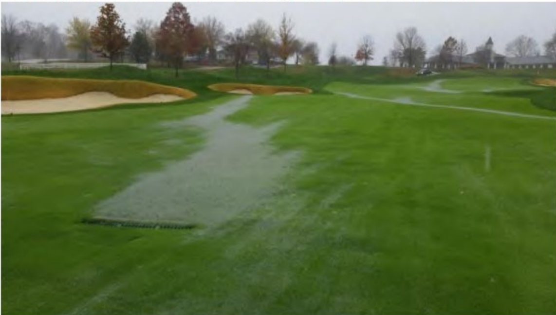
Figure 4- Channel Drain at Valhalla Golf Club
