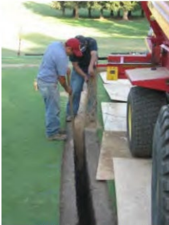
Backfilling trenching with sand
