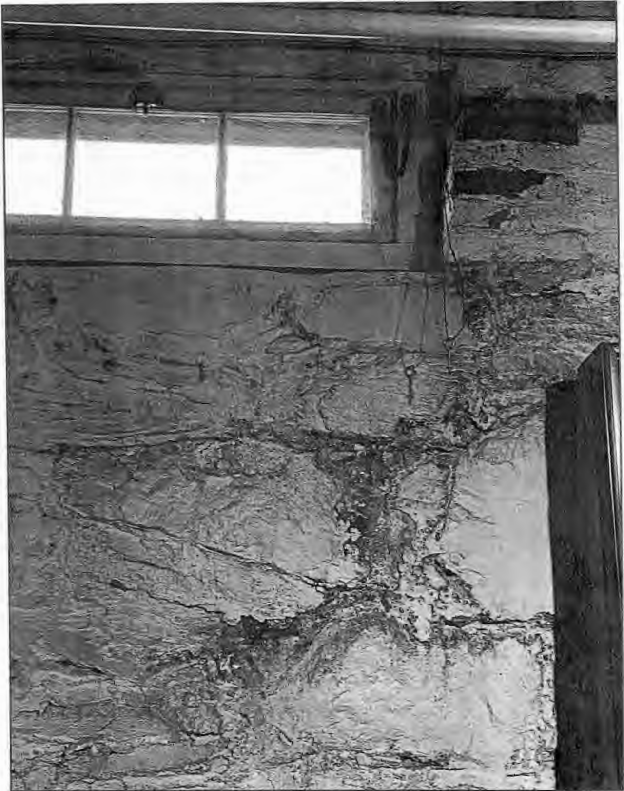
Foundation wall south
