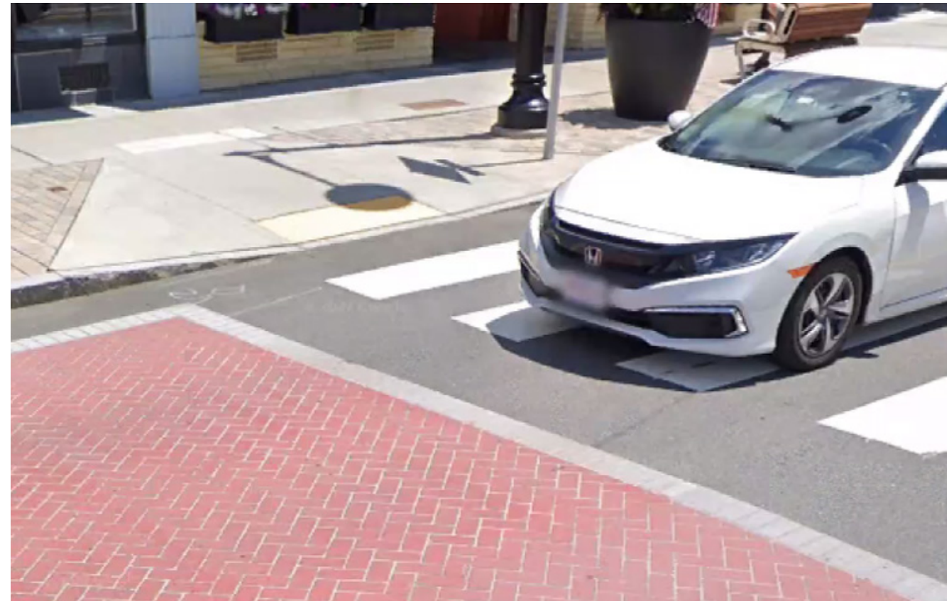
Beautification of pedestrian crossing at Walnut Street & Highland Ave
