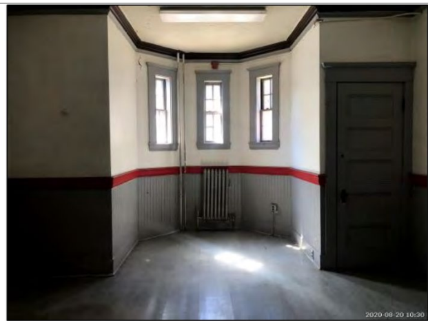
Photo 11: Ground level room, typical.
