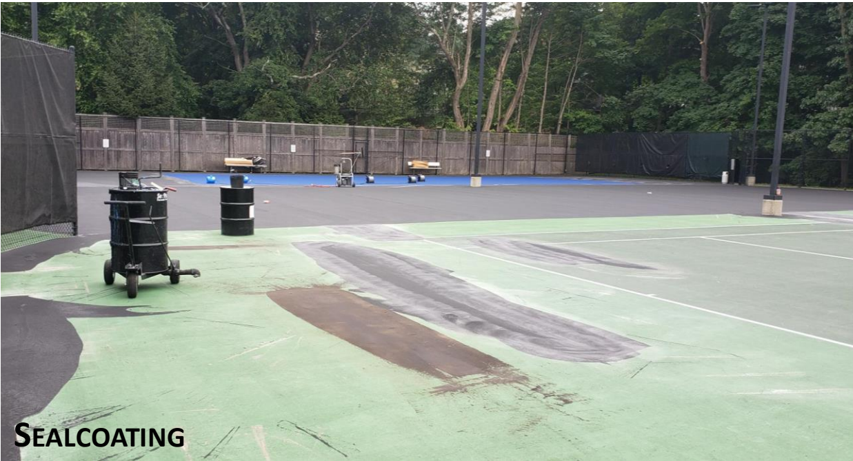
CRACK REPAIR MEMBRANE
