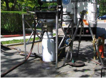
Installed cured-in-place liners in nearly 35,000 linear feet of old clay sewer main
