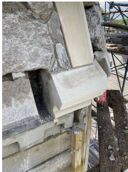
Existing and new masonry at base of spire was set in place and anchored to the inner masonry.
