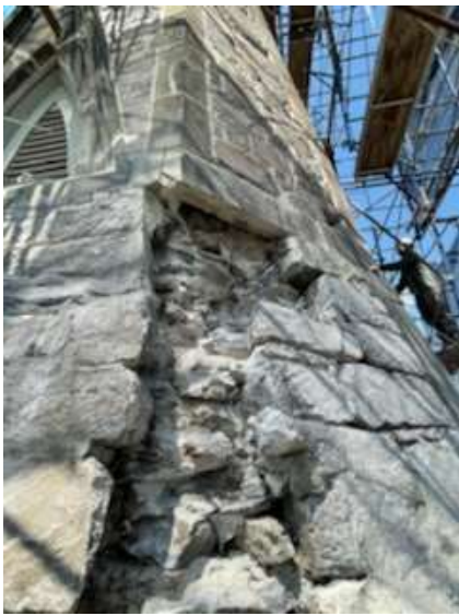
Loose exterior masonry at base of spire was removed to expose the inner masonry wall.
