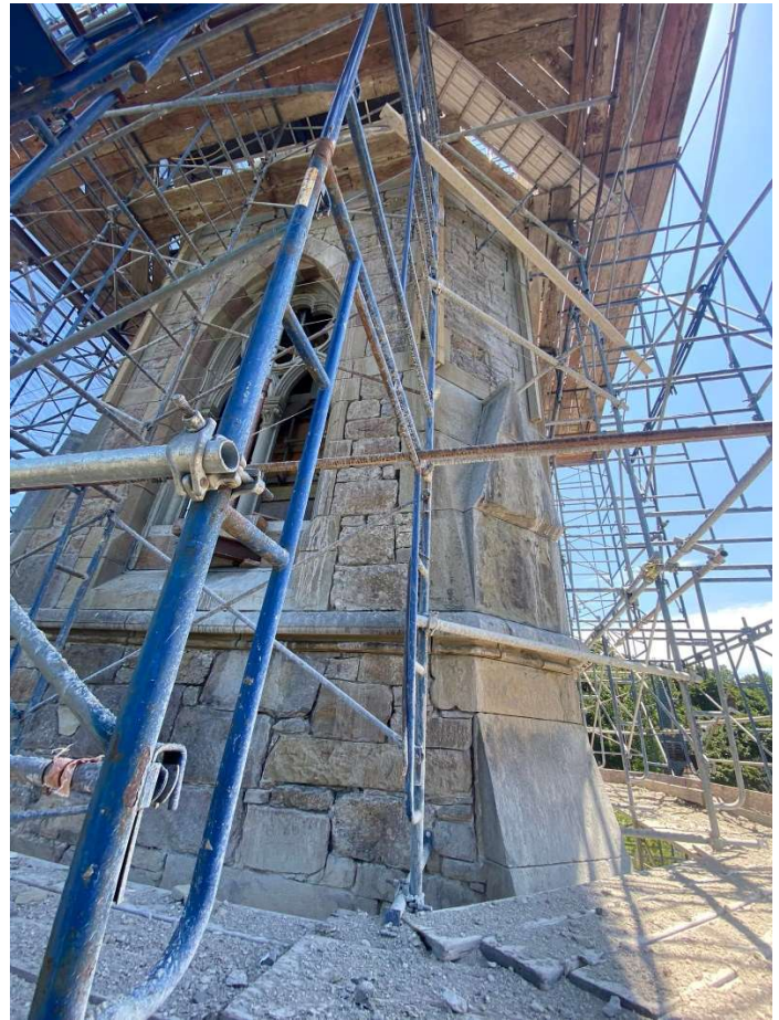
Next phase of work: pointing mid tower at Bell Loft
