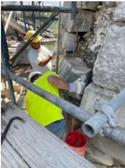
Existing and new masonry at base of spire was set in place and anchored to the inner masonry.
