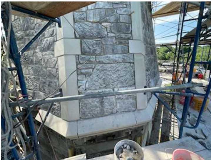
Reconstructed base of spire incorporated extensive areas of new material to replace fragmented stone.
