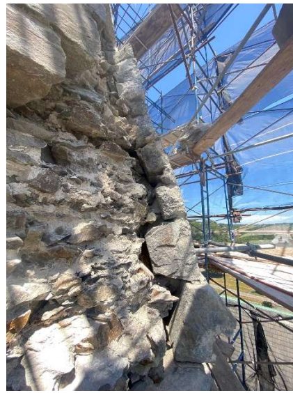
Loose exterior masonry at base of spire was removed to expose the inner masonry wall.
