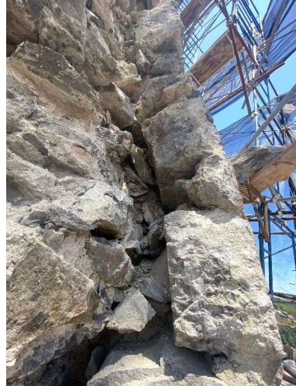
Loose exterior masonry at base of spire was removed to expose the inner masonry wall.
