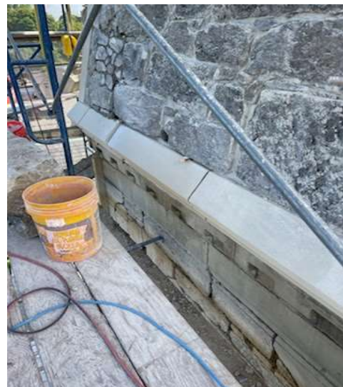
Reconstructed base of spire incorporated extensive areas of new material to replace fragmented stone.
