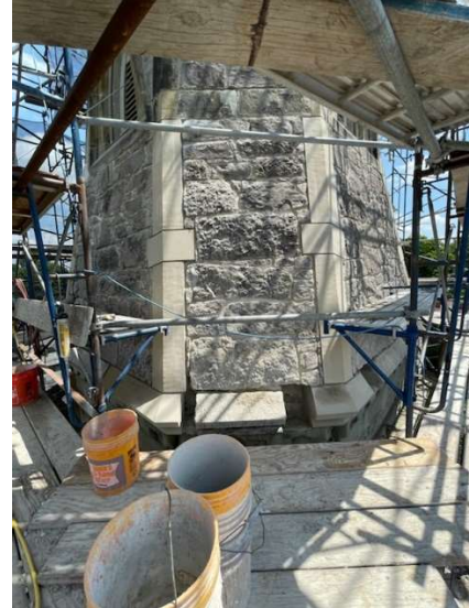
Existing and new masonry at base of spire was set in place and anchored to the inner masonry.
