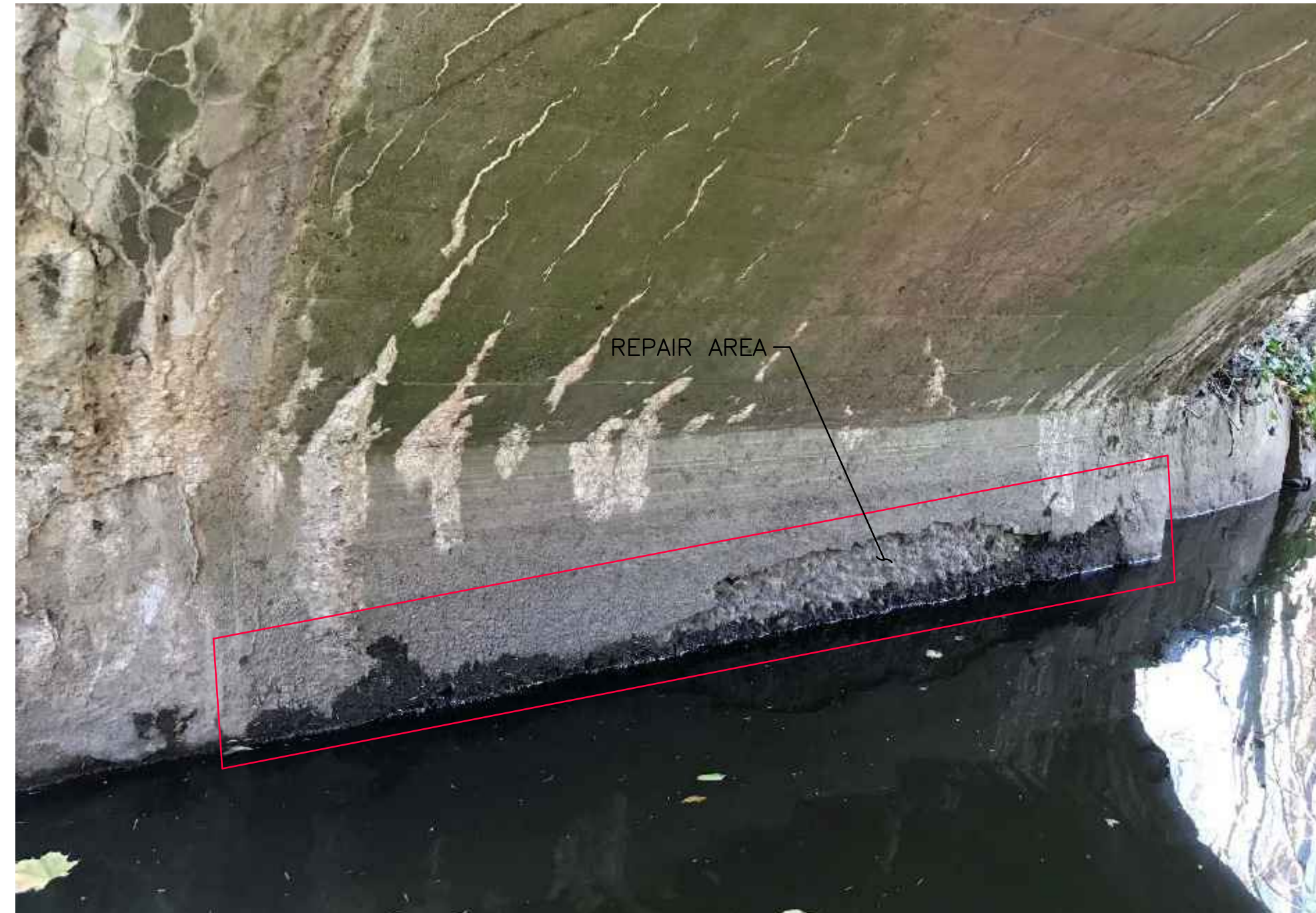
DOWNSTREAM BRIDGE – WEST ABUTMENT N.T.S.
