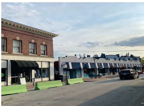
One and two-story retail in Newton Centre
