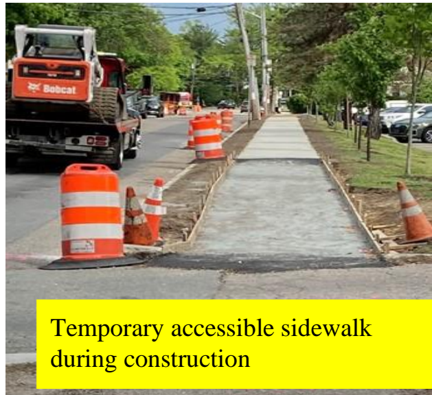
Temp. Asphalt ramp & temp cross walk painted
