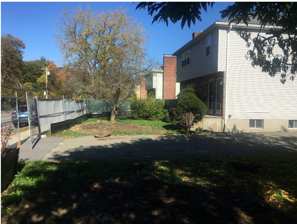
View to Northeast of Outer Buffer Zone on the Site showing Level Yard, Understory Tree, Paved Driveway, and Existing House and Construction Fence and Entrenched Silt Fence
