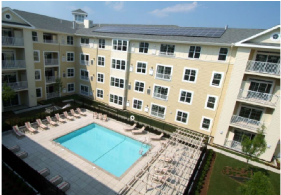
Parkside Commons Chelsea, MA (Solar Panels for energy management)
