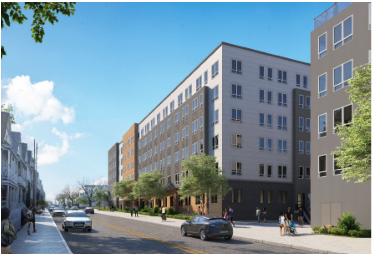
Innes Apartments, Chelsea MA - Under Construction
