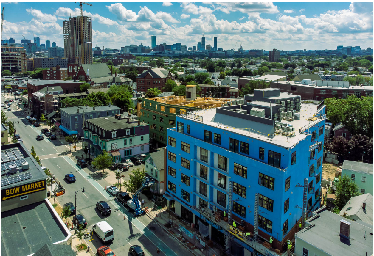
Union 346, Somerville, MA - Under Construction
