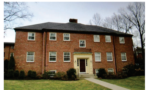
Multi-Family Residential: Garden Apartments 55-75 Wyman St, Waban Footprint: 2,200 sf
