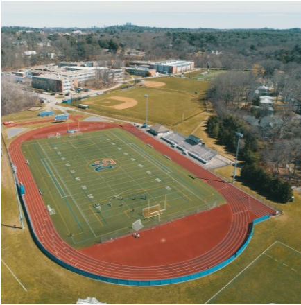
NSHS WINKLER STADIUM LIGHTS (2020)
