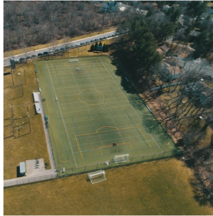
NSHS BRANDEIS RD FIELD LIGHTS (2022)
