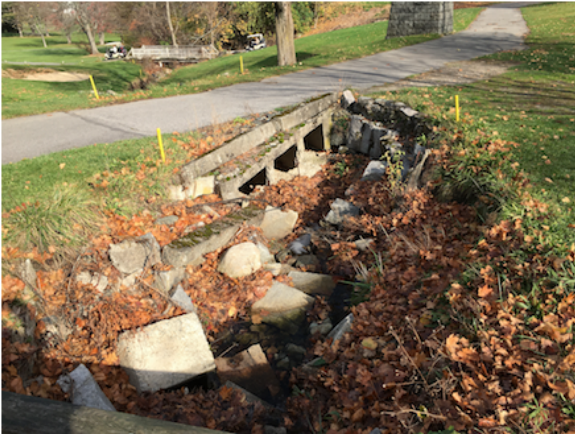
7 – culvert disrepair
