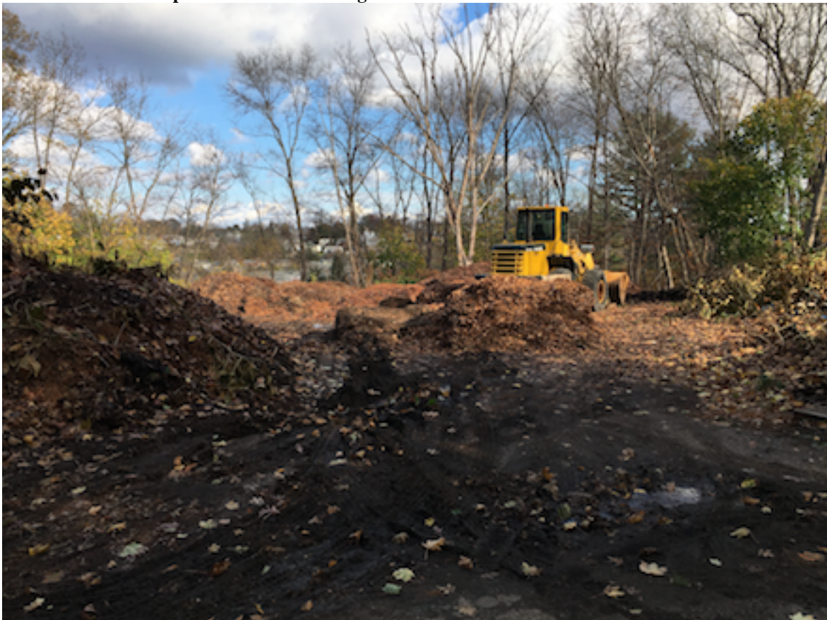
6 - Central debris dump filling up
