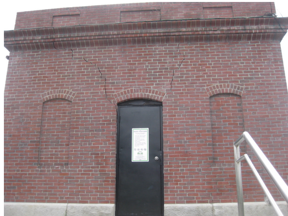
Waypoint 1: Clean looking gatehouse
