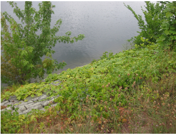
Waypoint 4: vines covering retaining wall
