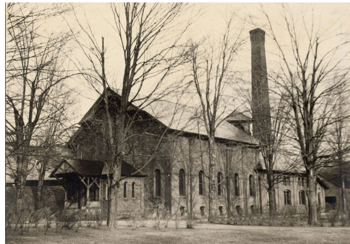
Newton Pumping Station - 1925
