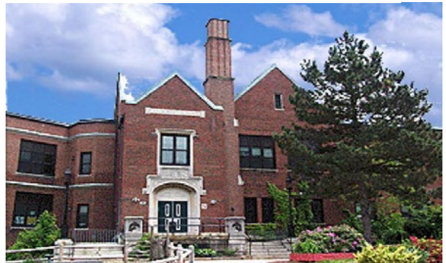
Ward Elementary School
