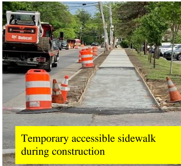
Temp. Asphalt ramp & temp cross walk painted
