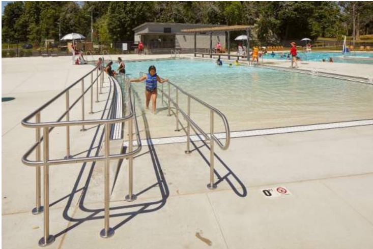
Ramp Access at Zero Depth Entry
