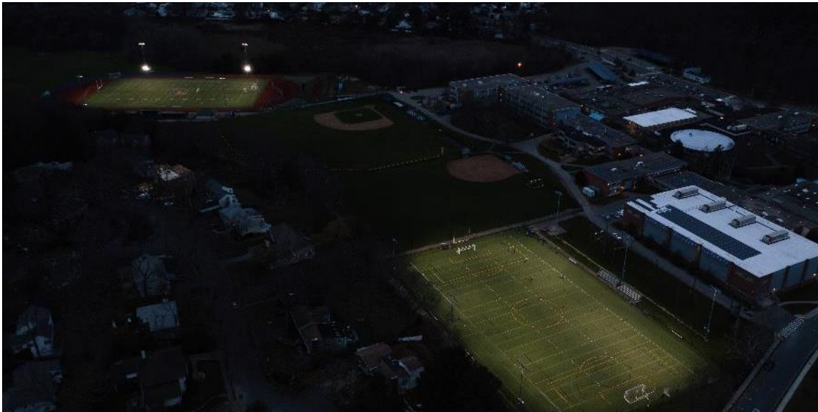
NSHS WINKLER STADIUM LIGHTS (COMPLETED)
