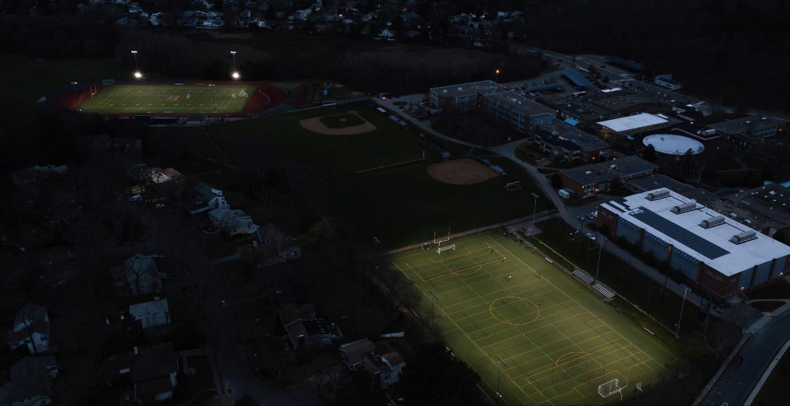
NEWTON SOUTH HIGH SCHOOL SPORTS LIGHTING
