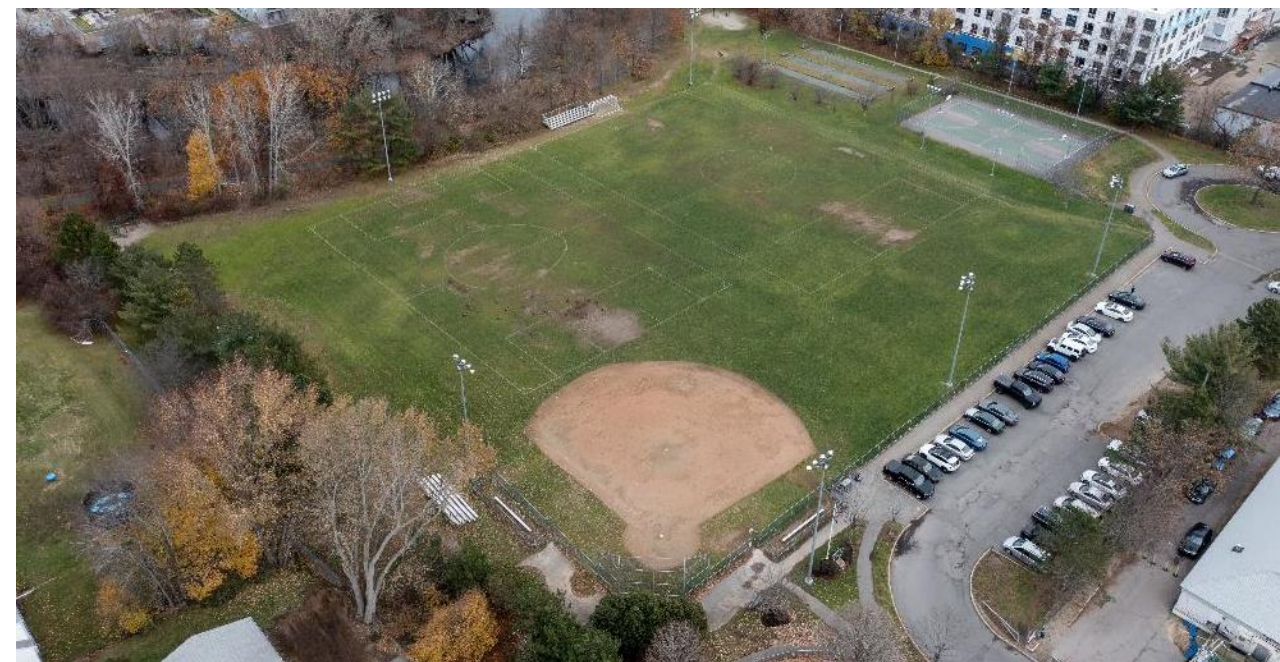
FORTE PARK MULTIPURPOSE SYNTHETIC TURF RETROFIT
