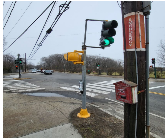
Pictured: Water ponding on the northwest corner of Crafts Street at North Street.
