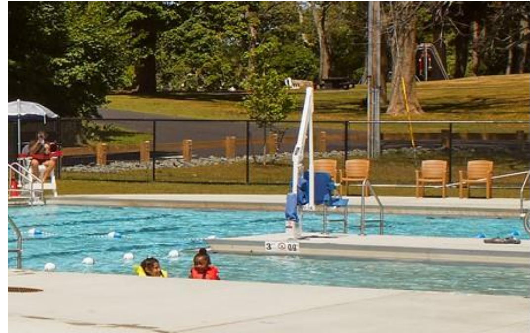
MAAB/ADA Compliant Pool Lift
