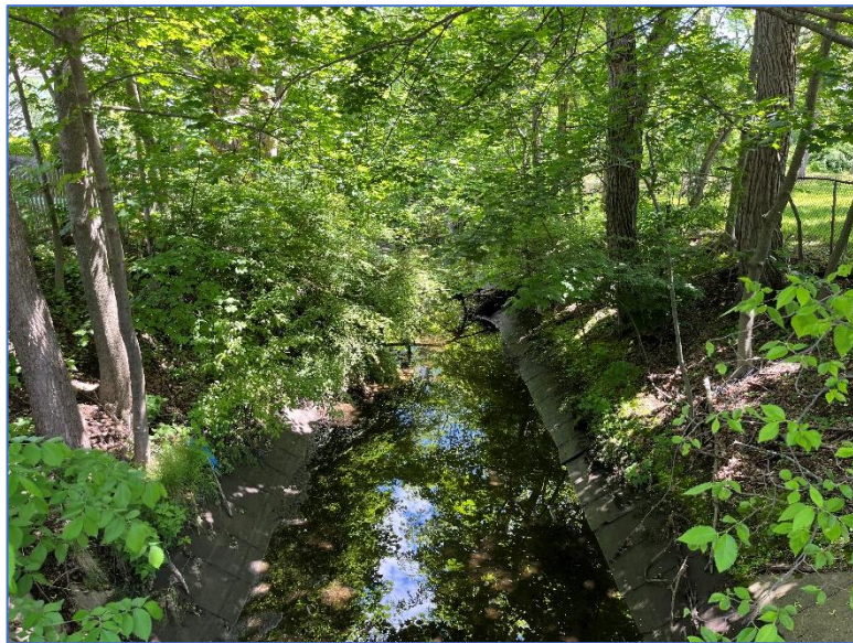
Photo 3. View of South Meadow Brook, which has been straightened and confined by retaining walls (Photo taken by HW in June 2022); additional photos of South Meadow Brook are provided in Attachment B.
