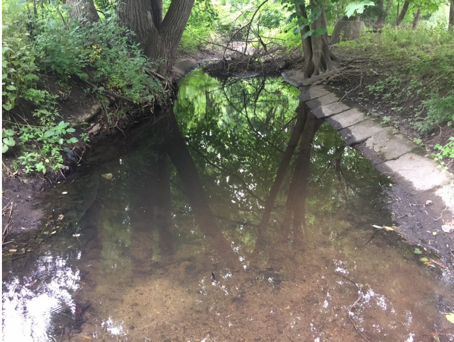
SOUTH MEADOW BROOK LOOKING UPSTREAM Note concrete lining at the base of the banks.
