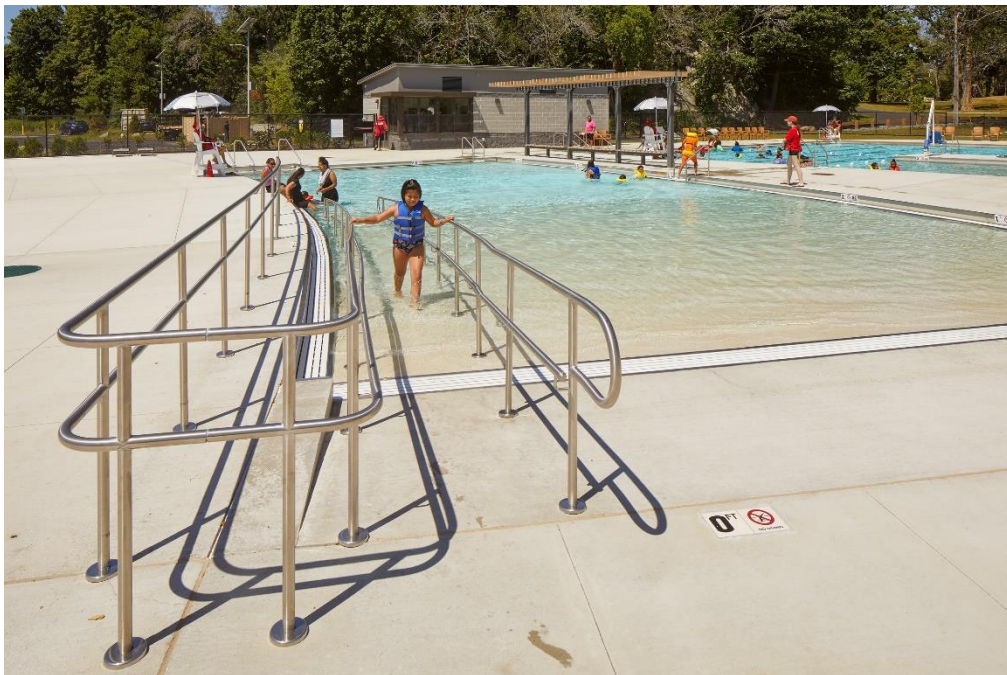
Ramp Access at Zero Depth Entry
