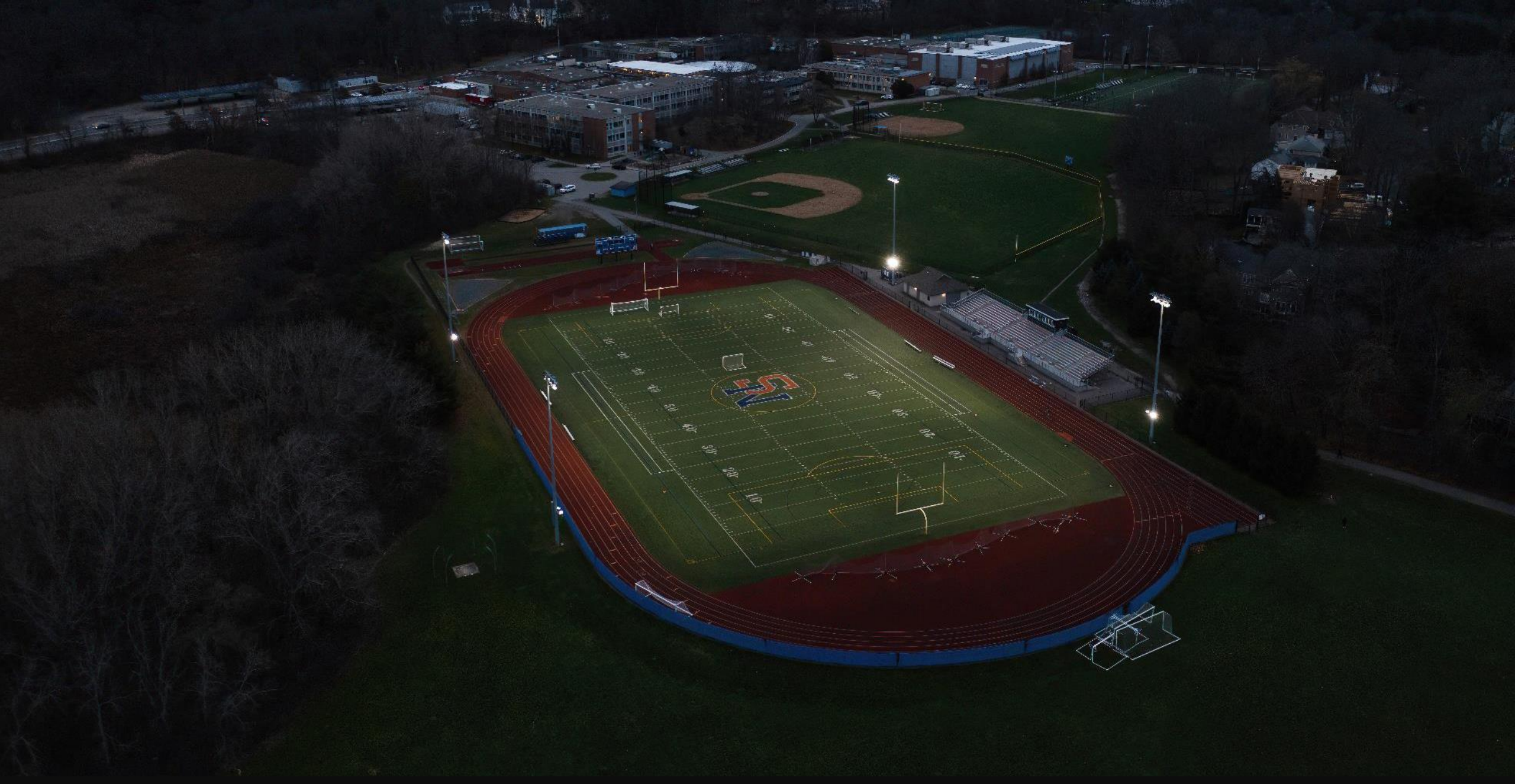
NEWTON SOUTH HIGH SCHOOL WINKLER STADIUM SPORTS LIGHTING
